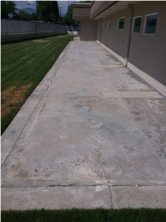
Concrete before project
