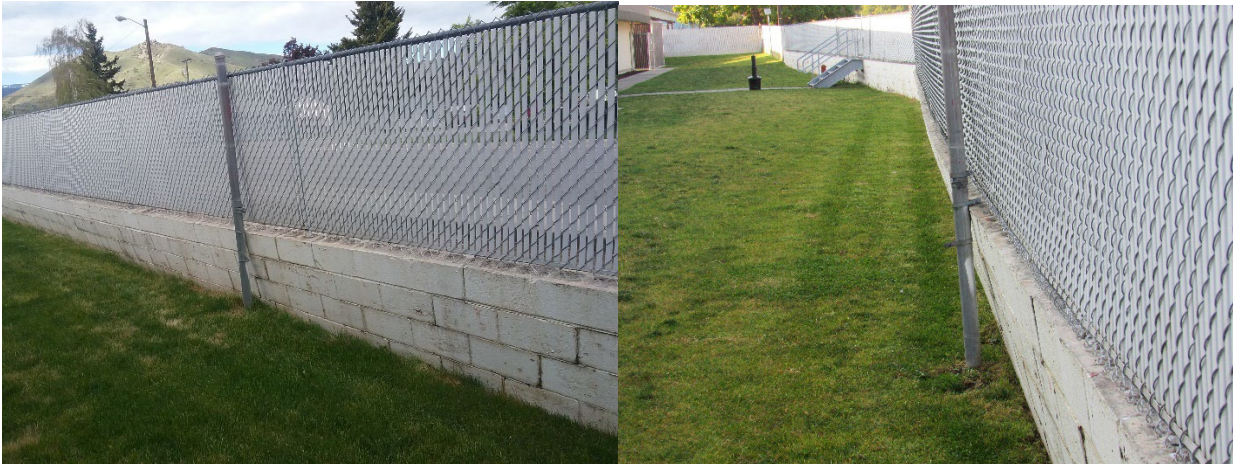
Retaining wall before project pictures
