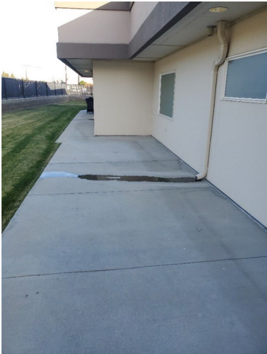
Concrete after project
