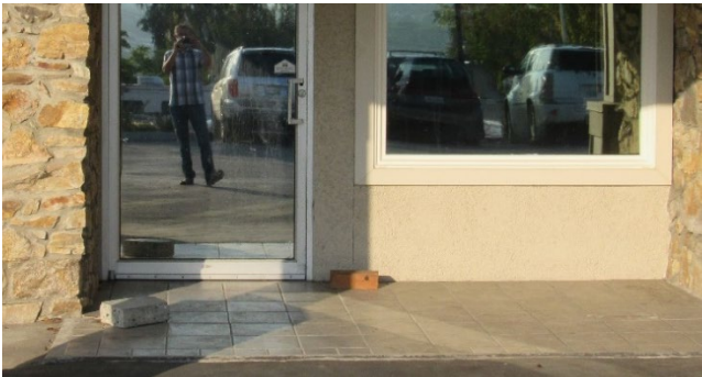
Entry C before project
