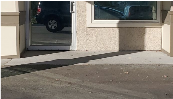
Entry C after project
