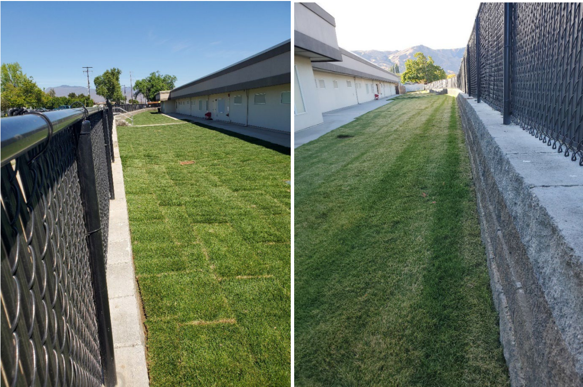
Retaining wall after project pictures
