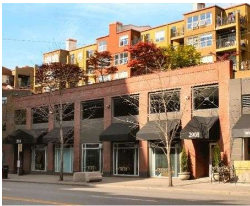
Figure E.8.1.b. This building uses openings on its second level parking area to resemble windows.
