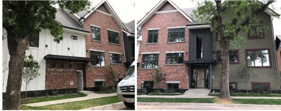
The above building uses fiber cement panels and planks in different textures and colors to help articulate the facade. The white color replicates the board and batten style in the left image and green color in the right image effectively replicates horizontal wood siding.
