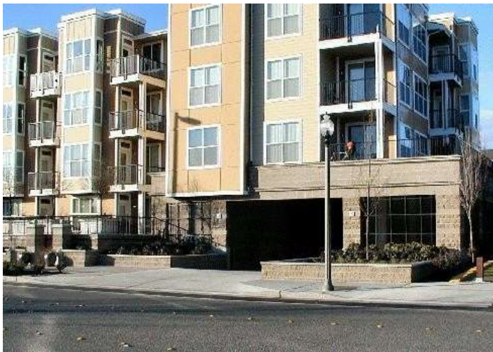
Figure E.8.1.c. Design parking garages to obscure the view of parked cars. Note the landscaping that separates the garage from pedestrians.
