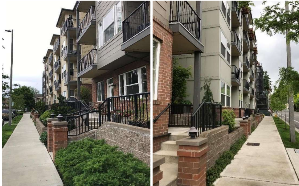
Figure C.1.c. The above images show ground-level residential frontages with setbacks of approximately 10 feet (left image) and 5 feet (right image) along different street frontages for this corner apartment building. These ground level units all have their own private unit access from the sidewalk and are elevated above the sidewalk to enhance the privacy to the units. The landscaping elements, brick posts, split-faced concrete block stoop walls, and black metal railings help to provide an attractive and effective transition between the public and private realm within the adjacent dwelling units.
