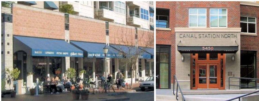
Figure E.6.1.b. The left facade illustrates an acceptable alternative example, as CMU is used as the primary cladding material. Note the use of split-facade CMU's above each of the awnings coupled with the use of smooth-facade CMU's on the vertical columns (which employ black accent tiles for added interest.). The right facade uses smooth-faced CMU for the main entry to function as a contrast to the brick (primary facade material) and to highlight the entry details (canopy, lighting, and doors).
