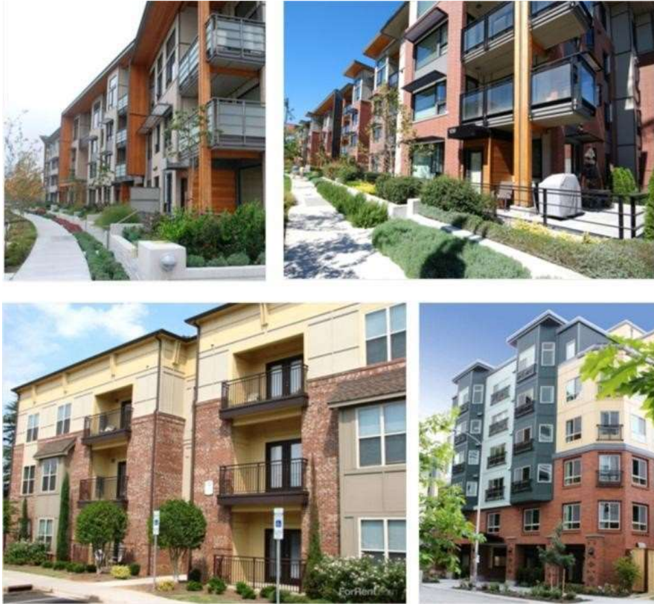
Figure E.3.1.e. Examples of articulation of multifamily residential building facades. All examples use window fenestration and vertical building modulation elements. The upper examples use a mixture of material changes and detail components to further articulate the facades. In the lower left example, the balcony element's dramatic mix of color, material, and projection are effective in meeting the standards. The lower right example adds a combination of materials, color changes, and building modulation to help meet the following standards.
