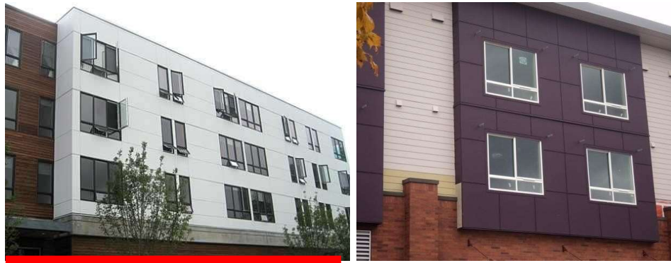
The fiber cement panels covering a large area in a single color would not meet the purpose of the standards. The right image is a better example and combines larger panels (dark maroon color) with horizontal planks (beige color) as effective articulation features.
