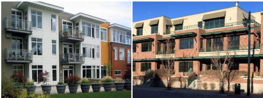
Figure E.3.1.g. Examples of acceptable vertical modulation. The example on the left features the stepping back of facade elements as well as different materials, colors and rooflines. In the example on the right, the balconies that have been integrated into the architecture of the building.
