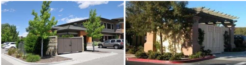
Figure C.7.2.a. Both examples use durable and attractive enclosures with trees and shrubs to soften views of the enclosures from the side. The right example uses a trellis structure on top – a desirable example particularly where the top of the enclosures are visible from surrounding buildings, streets, and pathways (due to topography or building heights).
