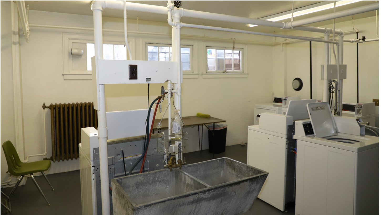
IMAGE 40. Before: 2020, basement, laundry room, looking southwest.
