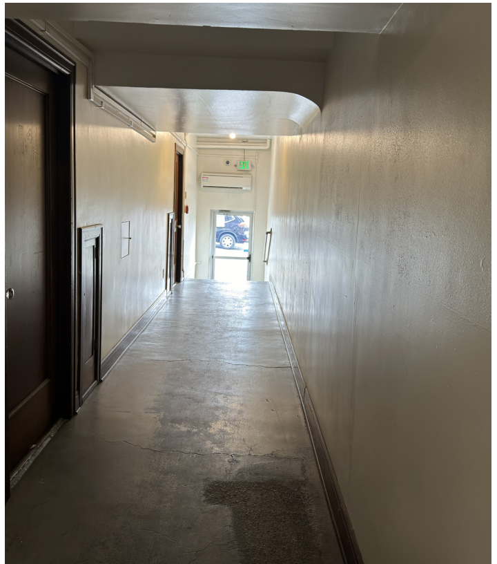
IMAGE 11. After: 2024, basement, hallway, looking north.
