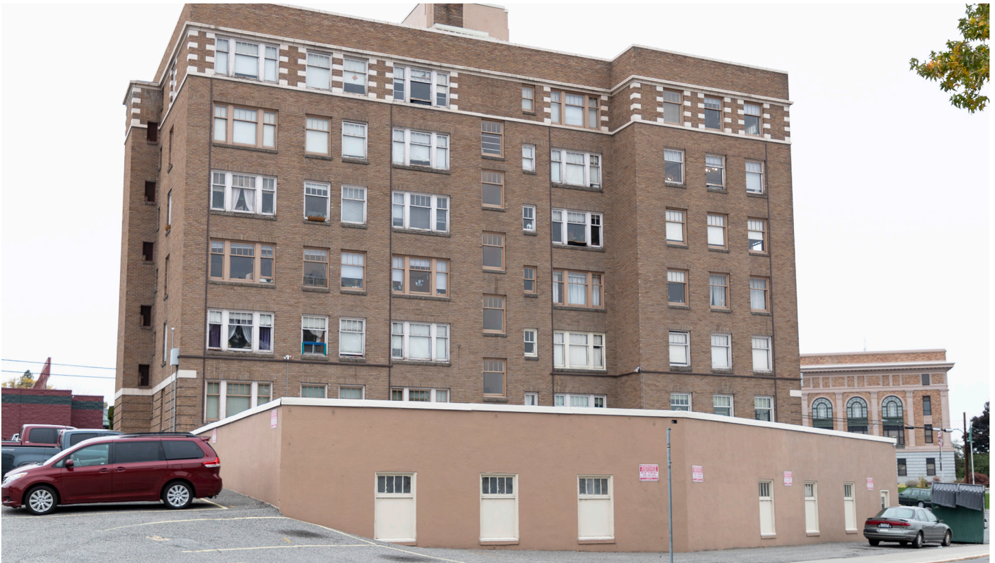
IMAGE 7. Before: 2020, exterior walls, east facade.
