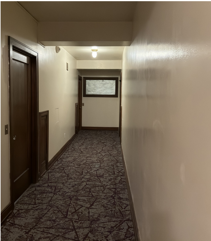
IMAGE 22. After: 2024, third floor, hallway, looking north.
