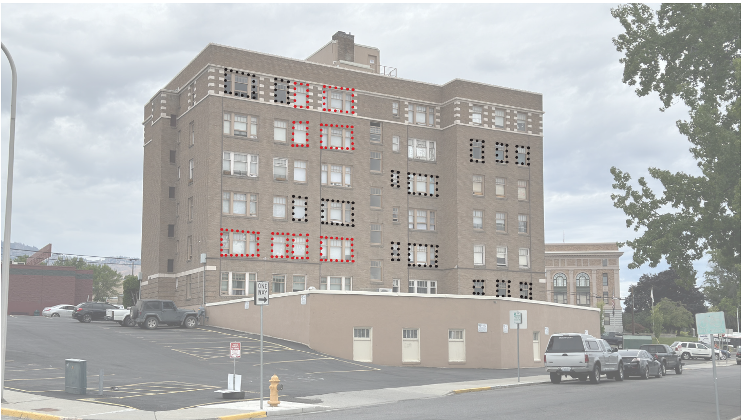
IMAGE 8. After: 2024, exterior walls, east facade. Repaired windows, black dots outline work completed in 2022; red dots outline work completed in 2024.
