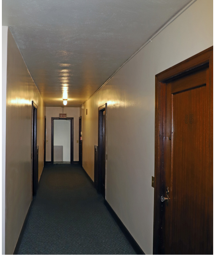
IMAGE 33. Before: 2020, sixth floor, hallway, looking south.
