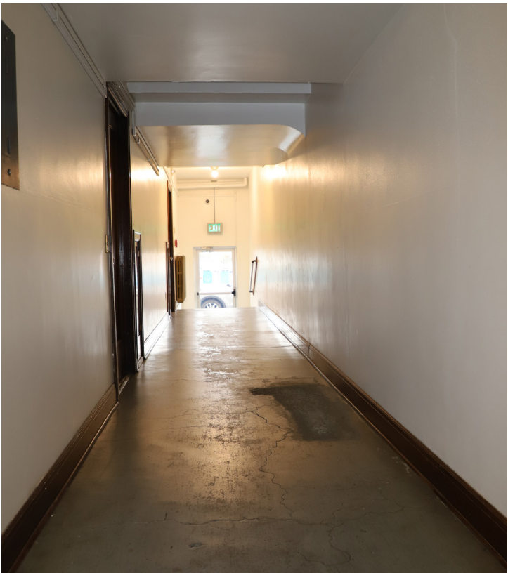
IMAGE 10. Before: 2020, basement, hallway, looking north.
