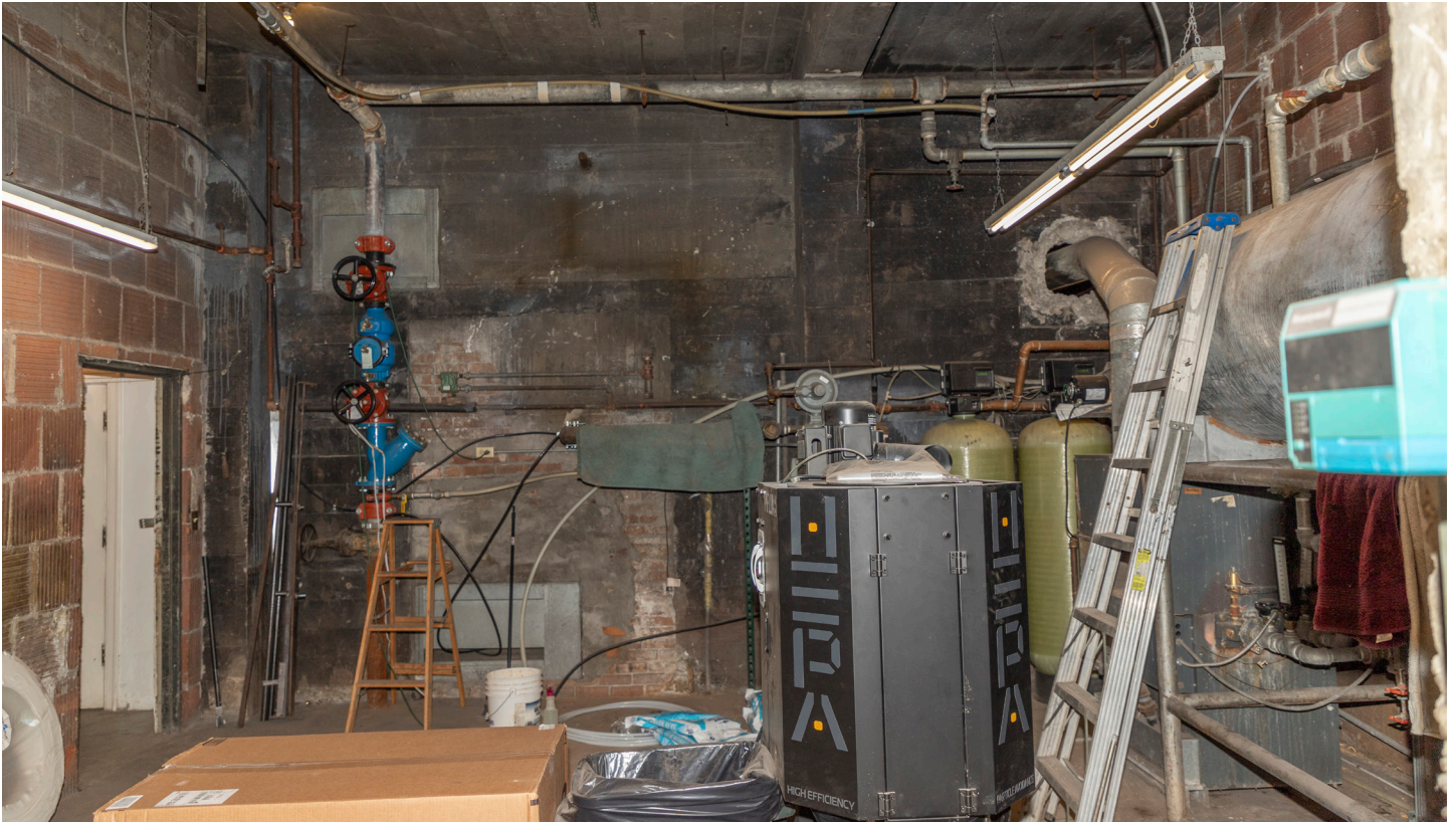
IMAGE 42. Before: 2022, basement, boiler room, east wall.
