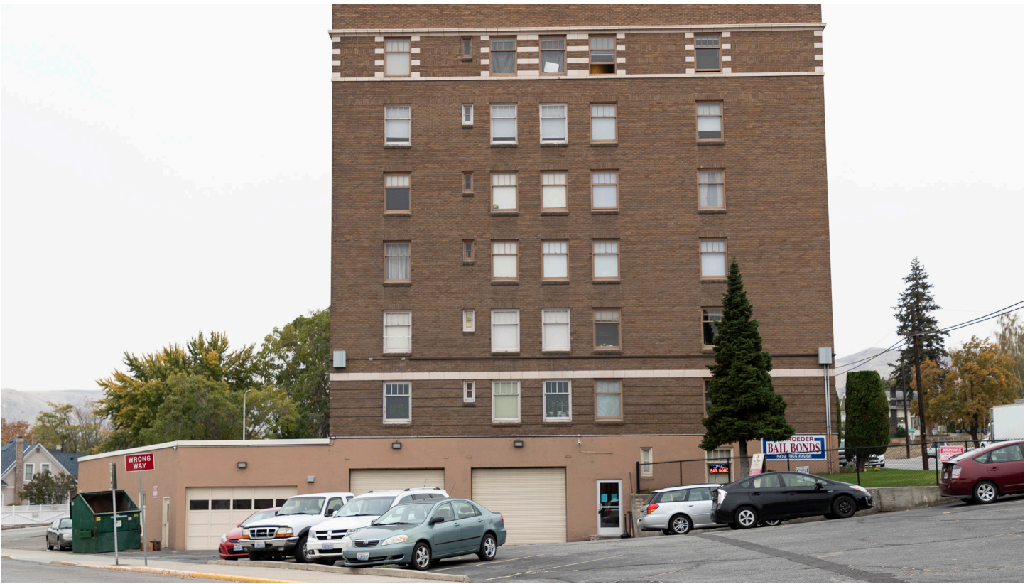
IMAGE 5. Before: 2020, exterior walls, north side facade.
