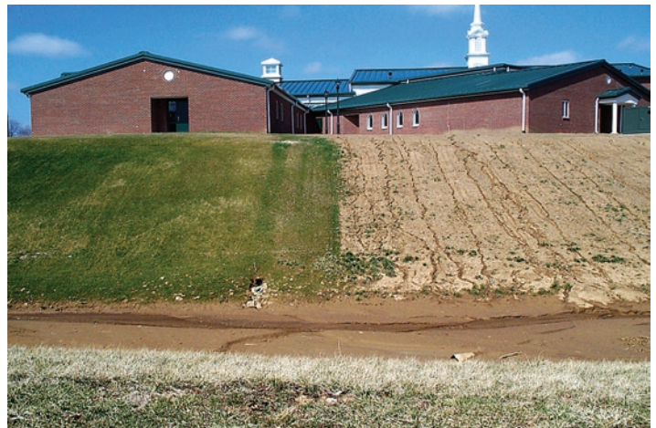
Figure 16. Seeding is an effective BMP that can be used to temporarily or permanently stabilize disturbed areas.
