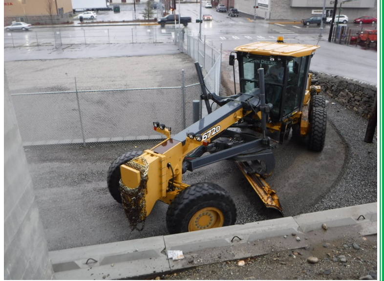
Picture 1: Alley Grading
