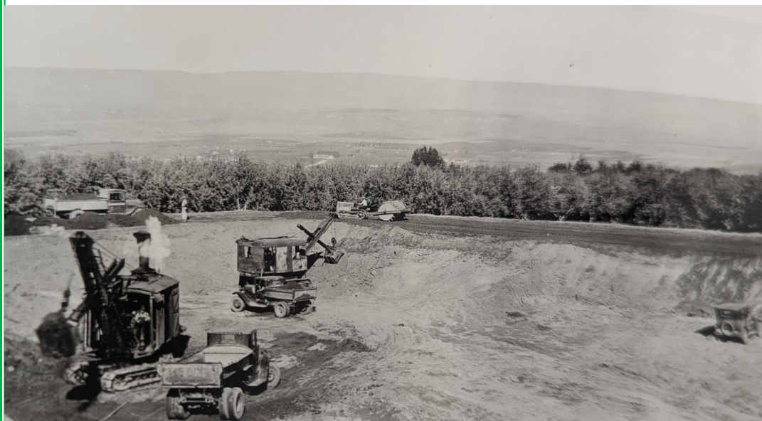
Picture 2: These photos were building the 4 Million Gallon Reservoir in 1931. You can see steam engines in use.
