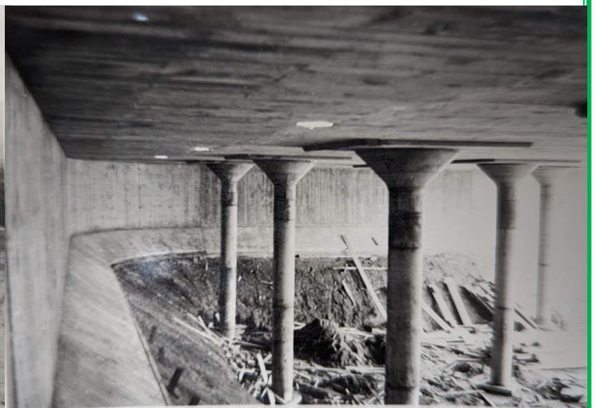
Picture 3: is the inside of the 4 Million Gallon Reservoir built in 1931. These are pillars similar to what is seen in the 8 mil reservoir.
