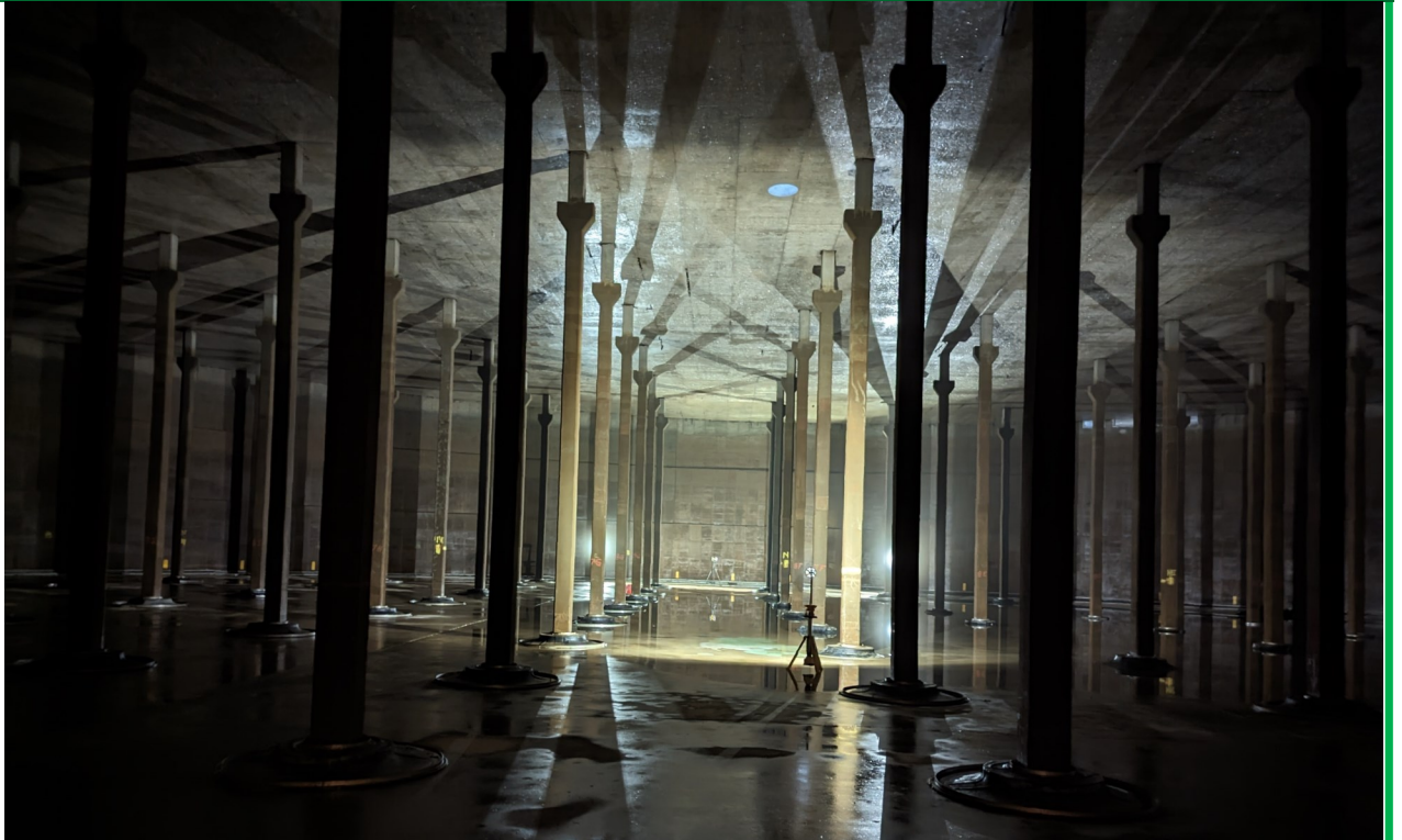
Picture 1: Inside the 8 Mil Reservoir, looking at some of the 109 pillars.
