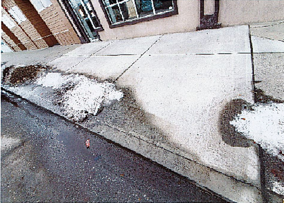
804 South Wenatchee after sidewalk replacement
