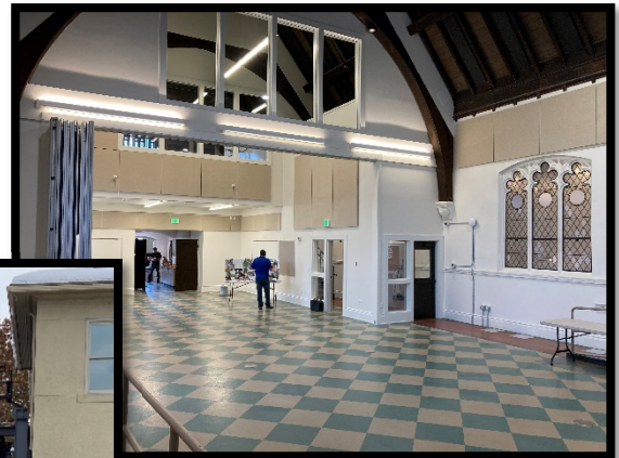
Above: Transformation of the Great Hall with a new operable wall, creating flexibility to the space.
