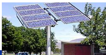
Pioneer Middle School Solar Panels
