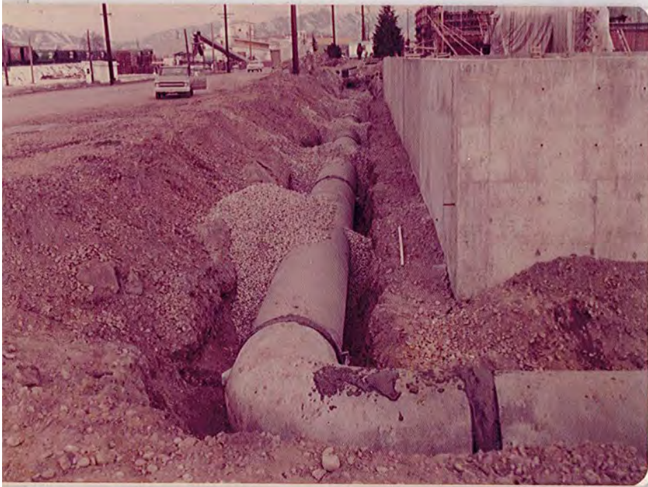
Primary Effluent Line Installation-Early 1970s
