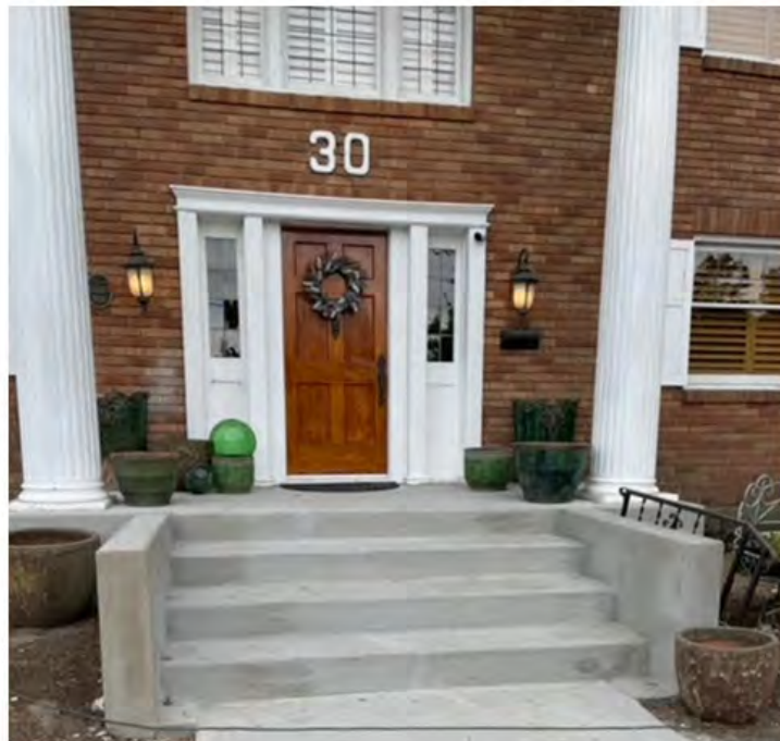
After modifications made to steps
