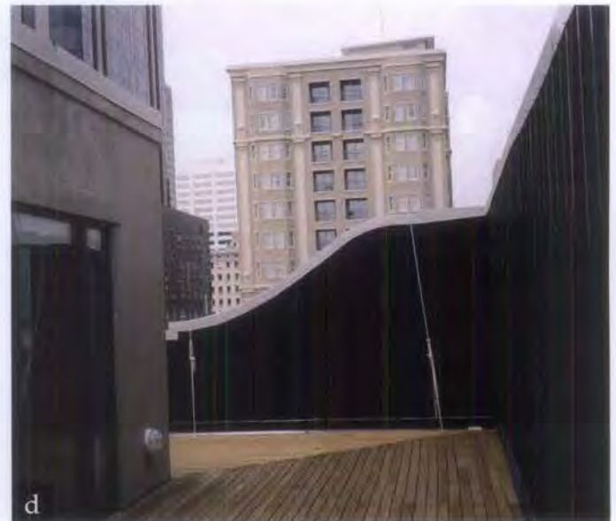
Figure 23. Colored flags marking the location of a proposed penthouse addition (a) were placed on the roof to help evaluate the impact and visibility of an addition planned for this historic furniture store (b). Based on this evaluation, the addition was constructed as proposed. It is minimally visible and compatible with the 1912 structure (c). The tall parapet wall conceals the addition from the street below (d).
