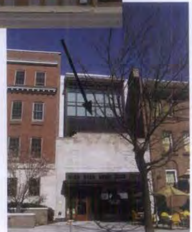
Figure 20. The height, as well as the design, of these two-story rooftop additions overwhelms the two-story and the one-story, low-rise historic buildings.
