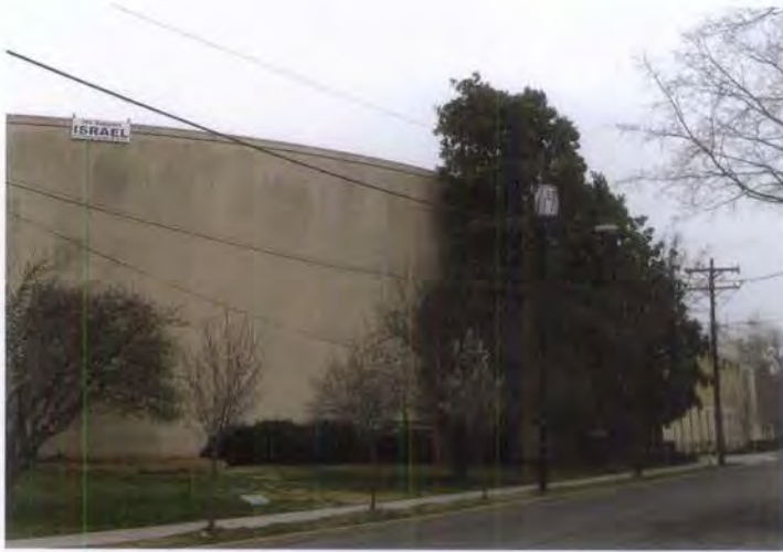
Figure 12. This 1954 synagogue (left) is accessed through a monumental entrance to the right. The new education wing (far right) added to it features the same vertical elements and color and, even though it is quite large, its smaller scale and height ensure that it is secondary to the historic resource.
