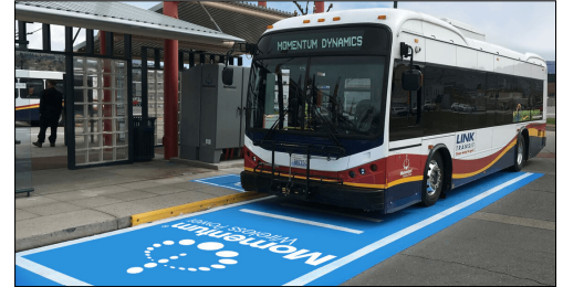
Wireless Inductive Bus Charger in Use
