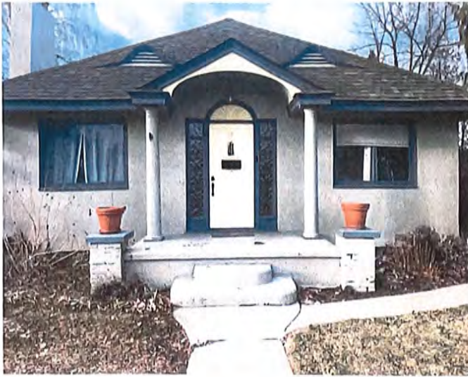
Photo of front of house from sidewalk. Picture windows to be replaced with similar picture windows. Wavy glass blocks to be replaced with picture windows. Front door to be replaced with something of similar style but in a new color to match the new paint choice. Mailbox to be fixed to house alongside front door. Window boxes to be added under existing picture windows and shutters to be added alongside windows (those features used to exist on the house).
