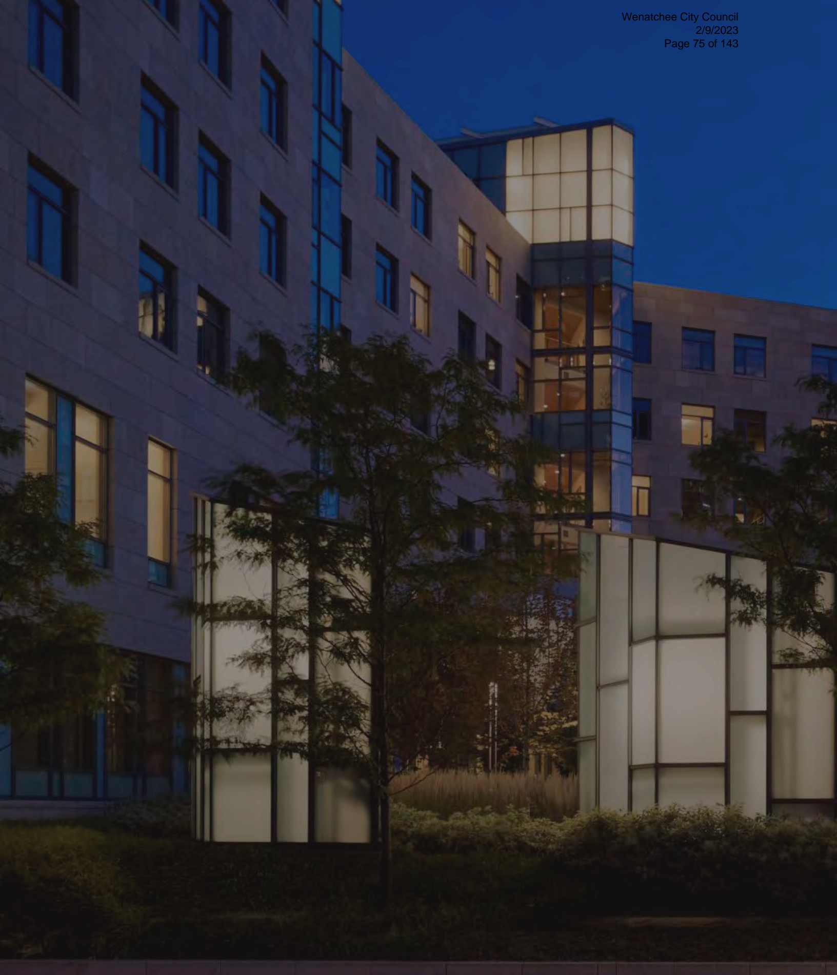
Streetscapes at the MIT Sloan School of Management are performative, with light monitors functioning as exhaust for the building's underground parking garage - promoting pedestrian safety and art at the same time. Cambridge, MA, David Cutler with Moore Ruble Yudell and Halvorson Landscape Architects
