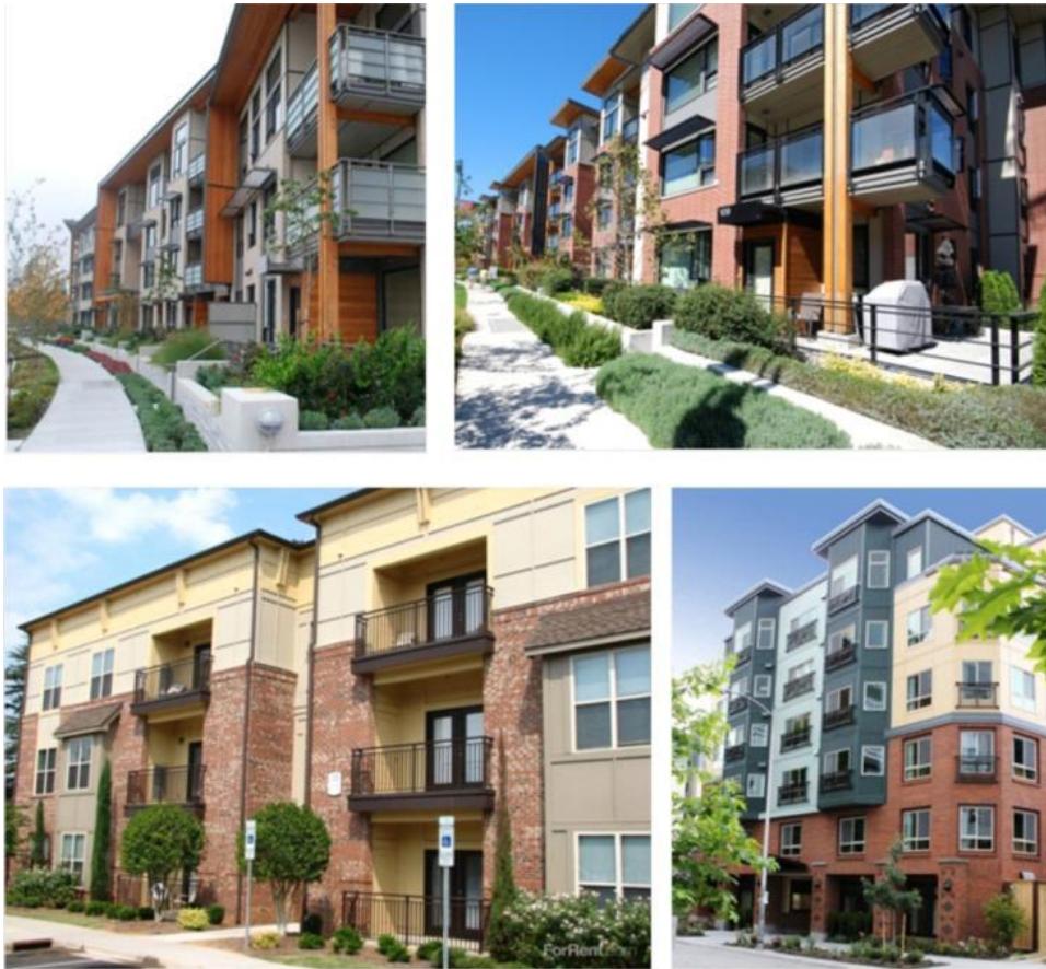
Figure E.3.1.e. Examples of articulation of multifamily residential building façades. All examples use window fenestration and vertical building modulation elements. The upper examples use a mixture of material changes and detail components to further articulate the façades. In the lower left example, the balcony element’s dramatic mix of color, material, and projection are effective in meeting the standards. The lower right example adds a combination of materials, color changes, and building modulation to help meet the following standards.
