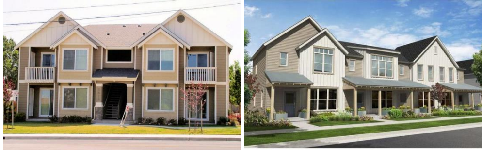
Figure E.3.1.b. Two examples of modulation effectively used on a duplex (left) and a triplex (right).
