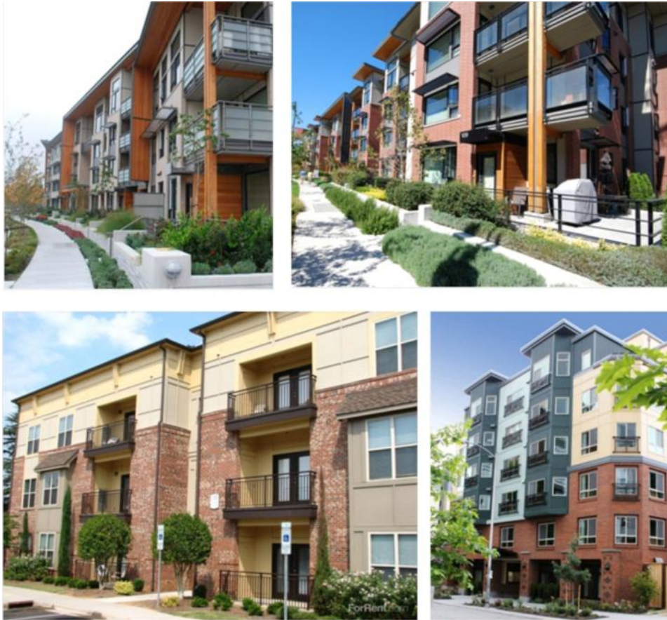
Figure E.3.1.e. Examples of articulation of multifamily residential building façades. All examples use window fenestration and vertical building modulation elements. The upper examples use a mixture of material changes and detail components to further articulate the façades. In the lower left example, the balcony element's dramatic mix of color, material, and projection are effective in meeting the standards. The lower right example adds a combination of materials, color changes, and building modulation to help meet the following standards.
