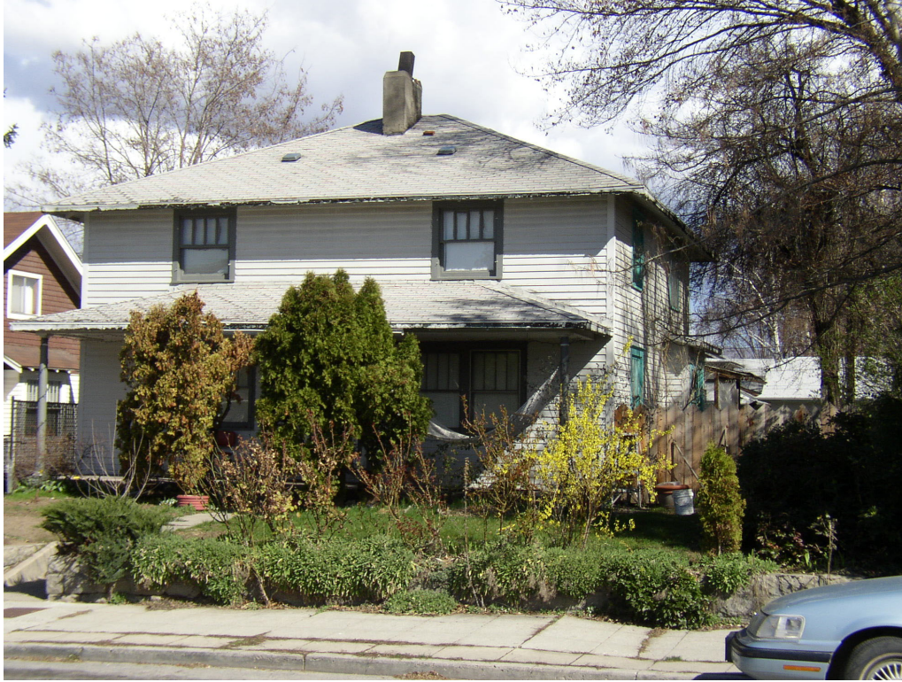
Photo 3 – Inventory photo for 151 S. Emerson window showing south façade visible
