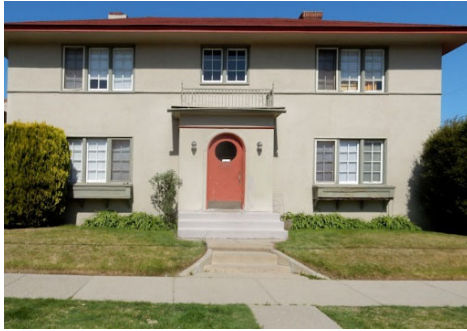
Figure E.3.1.f. This handsome house in a Core Residential Character Area uses window patterns and planter boxes as well as an entry feature to articulate its façade, rather than modulation and material changes.
