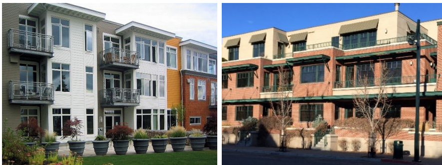
Figure E.3.1.g. Examples of acceptable vertical modulation. The example on the left features the stepping back of façade elements as well as different materials, colors and rooflines. In the example on the right, the balconies that have been integrated into the architecture of the building.
