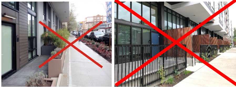
Figure C.1.d. Ground floor residential units such as these often lack privacy and the livability of outdoor spaces is limited. Locating the ground floor at or close to grade or with insufficient setback results in an uninviting space even with the planter in place. This condition should be avoided.
