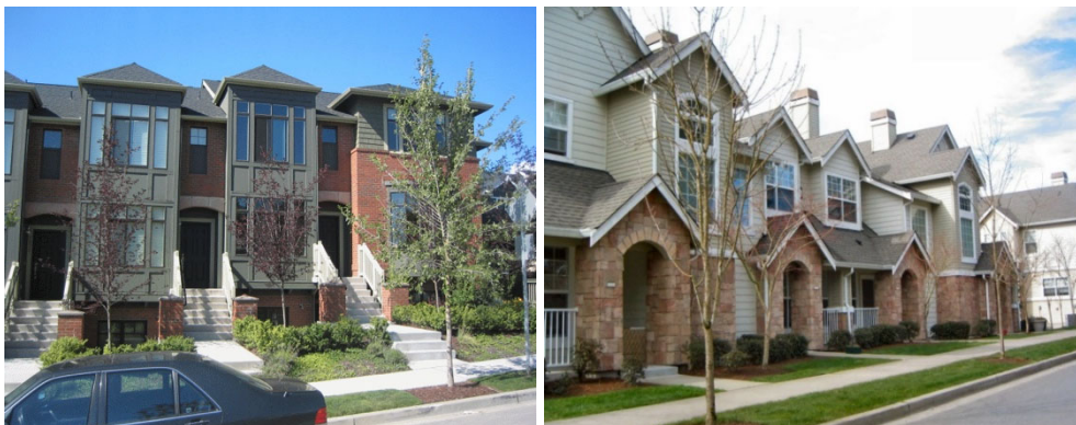
Figure E.3.1.c. The units in the left image each have distinct, but identical windows and roof forms. The outside unit on the right is differentiated through the use of
