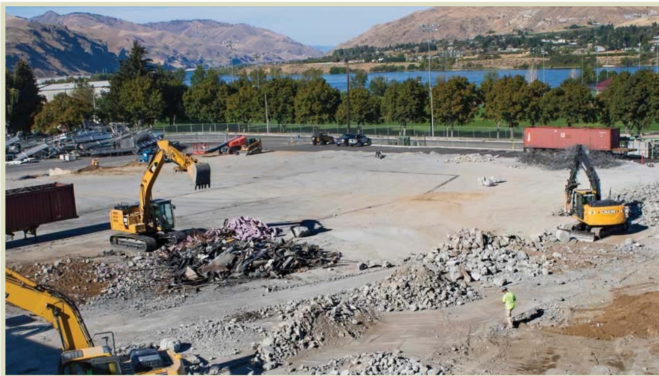
Workers break up concrete from a Blue Bird Inc. warehouse that was destroyed by a wildfire to prepare the site for construction in Wenatchee, Washington on September 9, 2015.
