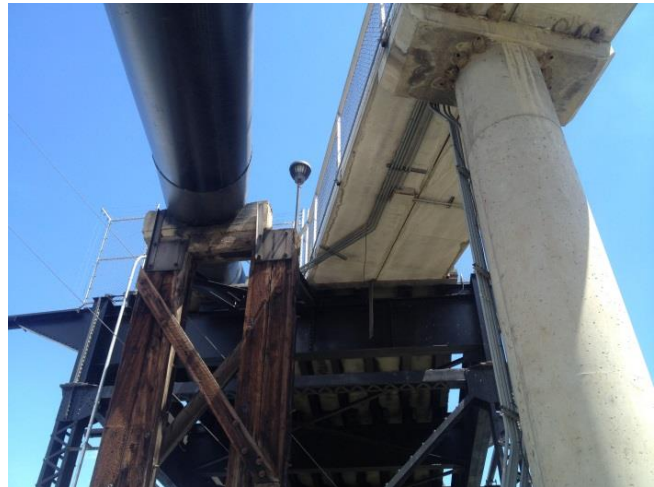
Western Terminus of Existing Pedestrian Bridge
