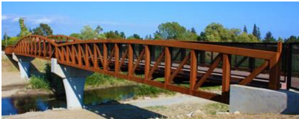
Example of a Weathering Steel Bridge
