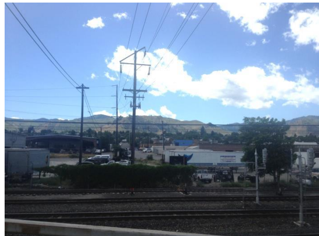
View Looking West From the Existing Ped Bridge
