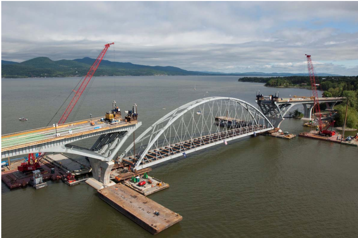
Figure 4: Example of Pre-assembly Erection of Tied Arch Bridge
