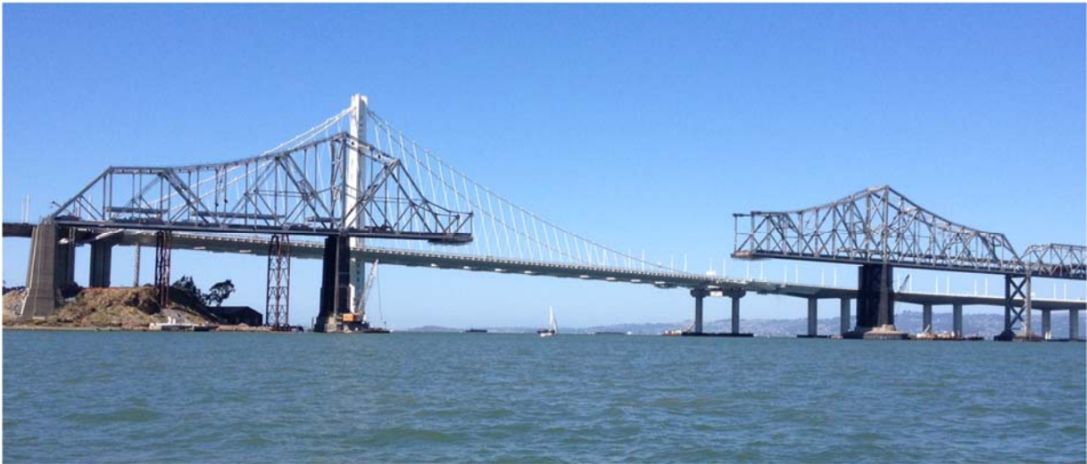
Figure 5: Example of Cantilever Truss Bridge Construction
