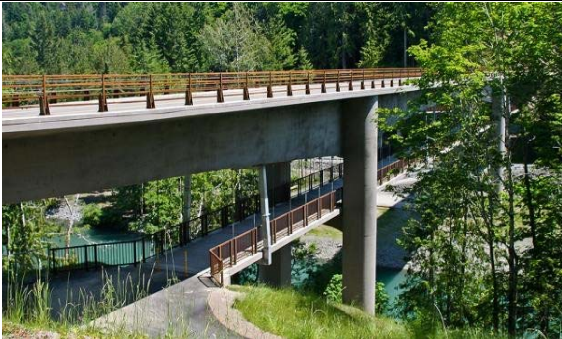
Figure 7: Suspended Pedestrian Structure Below Elwha River Bridge
