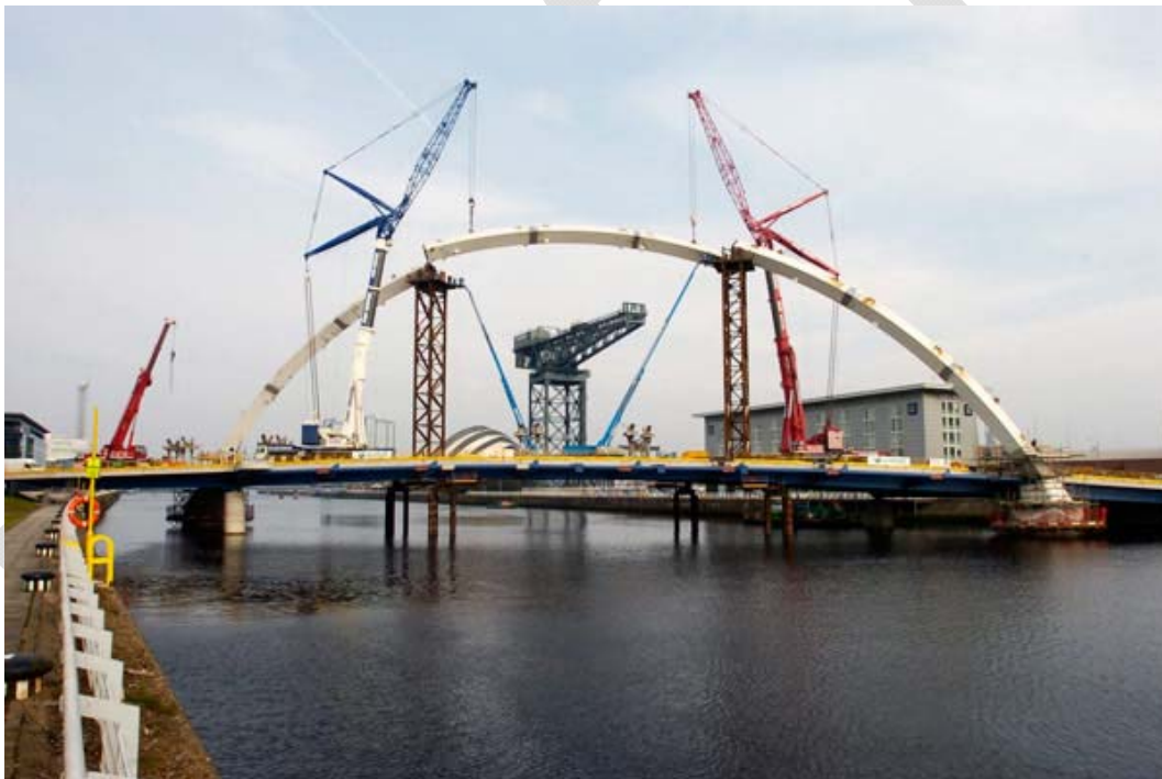
Figure 3: Example of In-Situ Tied Arch Bridge Construction
