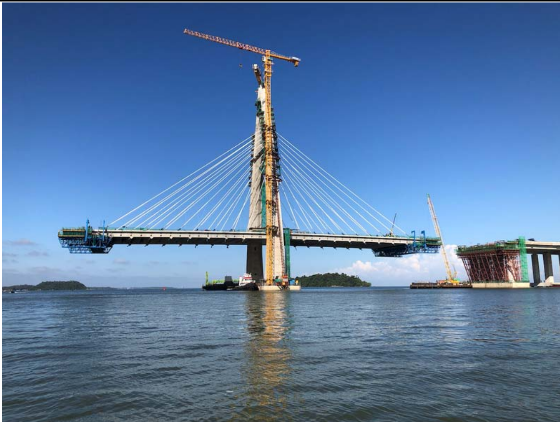
Figure 6: Example of Cable-Stayed Bridge Construction
