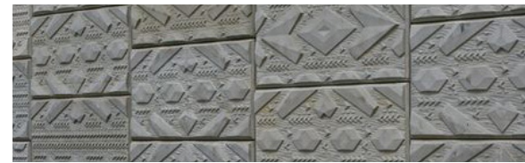
Custom Wall Finishes
