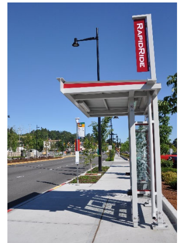
Bus Transit Facility, Rainier Avenue S (SR 167) Improvements, Renton
