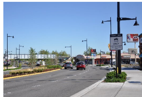
Driveway Entrance, Rainier Avenue S (SR 167) Improvements, Renton
