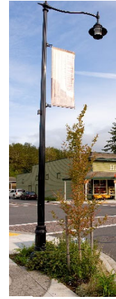
Decorative Illumination Pole, Town Center Improvements, Snoqualmie
