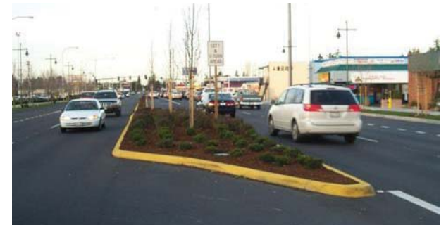
EXAMPLE: U-Turn Median Pocket. Seattle, WA (above two) (image: Federal Highway Administration)
