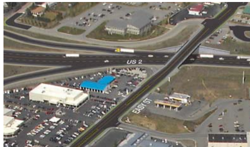
Easy Street crossing over US 2 allows safer, more efficient connectivity for local traffic
