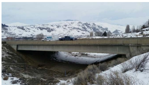
Existing Underpass to be Used to Replace Existing At-Grade Intersection
