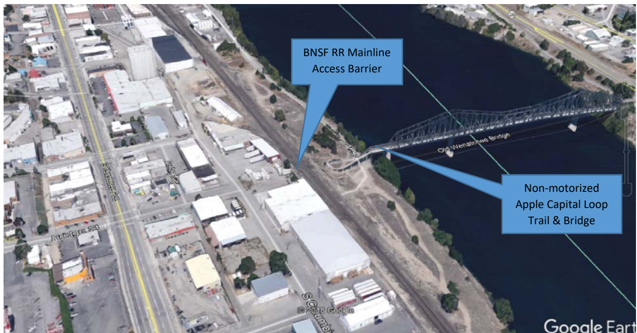
Existing Pedestrian Barrier
