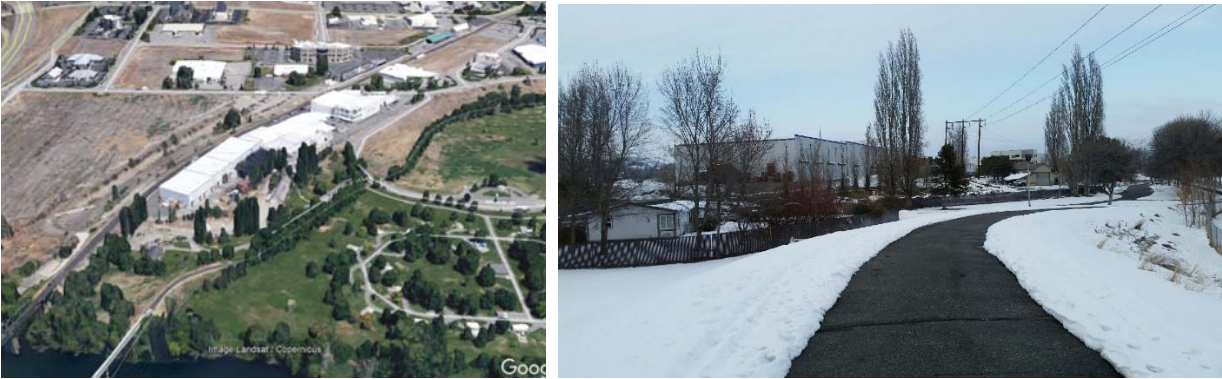
Confluence Parkway Along Edge of Park and Industrial Area
