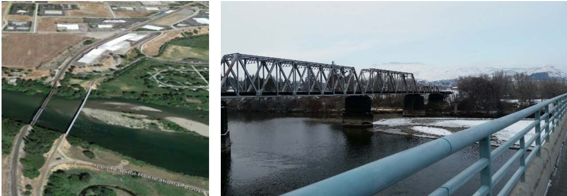
Confluence Parkway River Crossing - Between BNSF Shortline and Non-Motorized Trail Bridges
