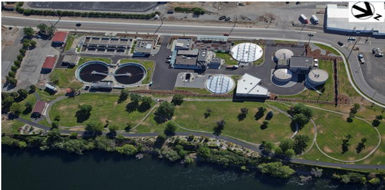
Photo credit: Jacobs Engineering 2022
