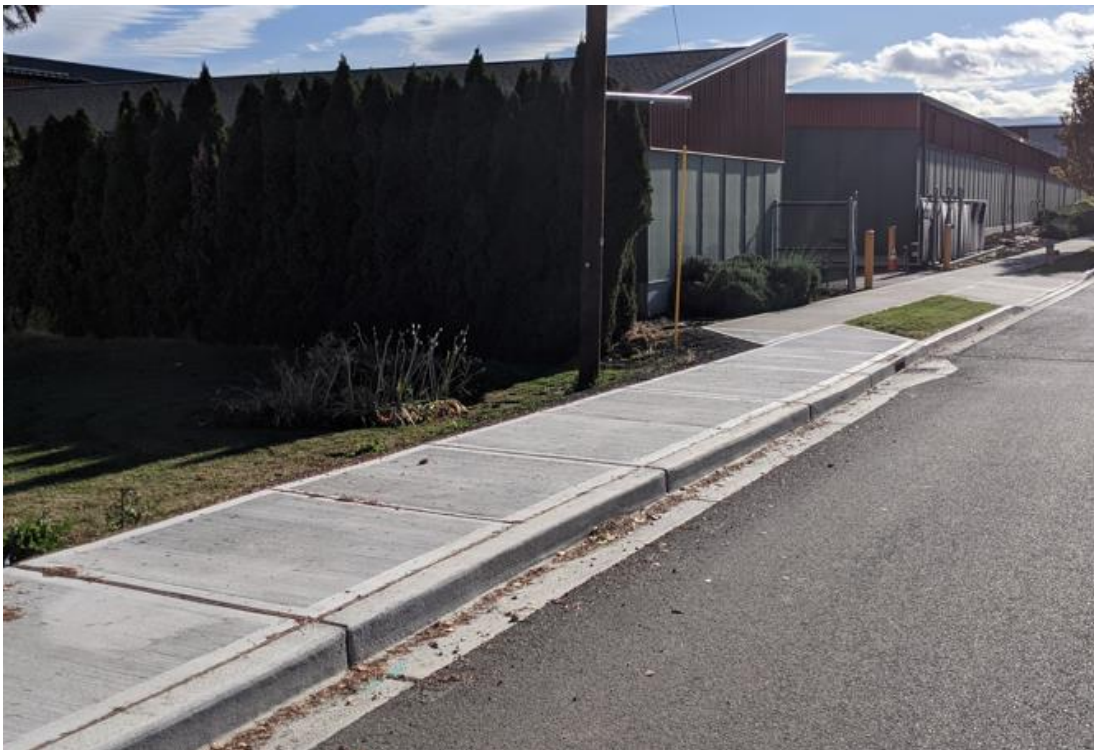
New sidewalk, looking South on Stella St.
