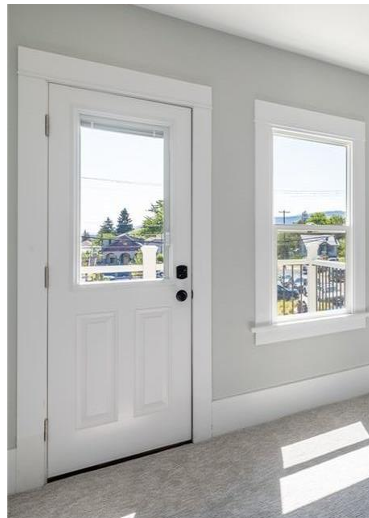
Balcony Door After
