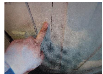
Basement Door Before
