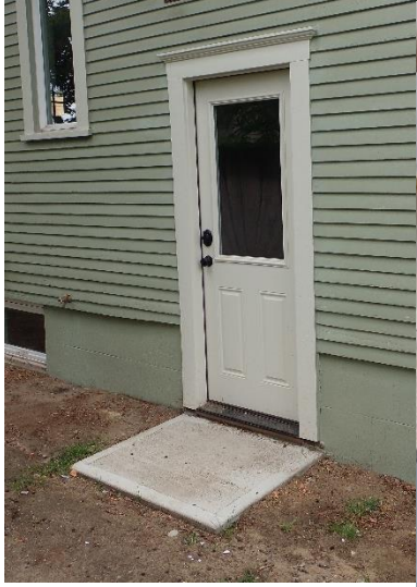
Basement Door After
