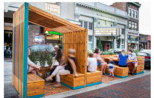
Coated wood planters as barrier walls
