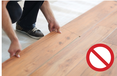
Interior laminate flooring is not acceptable
