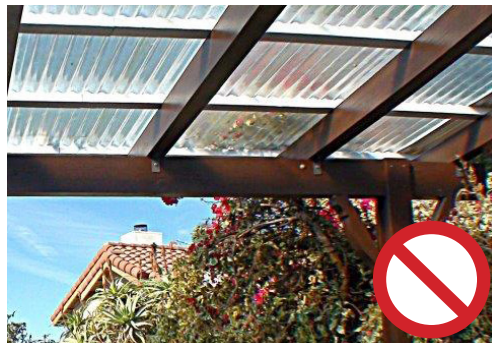
Corrugated plastic is not acceptable
