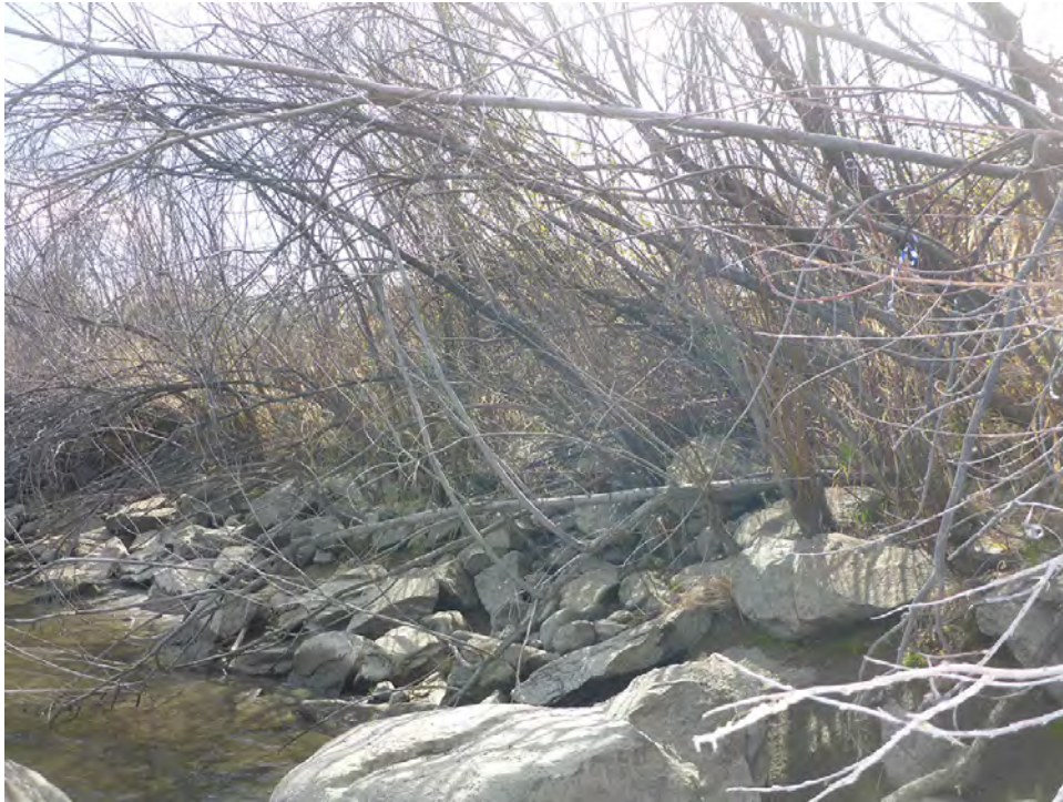
Photograph 17 Bank Armoring along Right Bank of Wenatchee River
