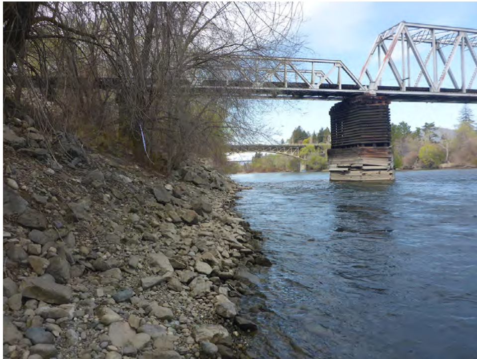
Photograph 5 Wenatchee River Right Bank (looking upstream)
