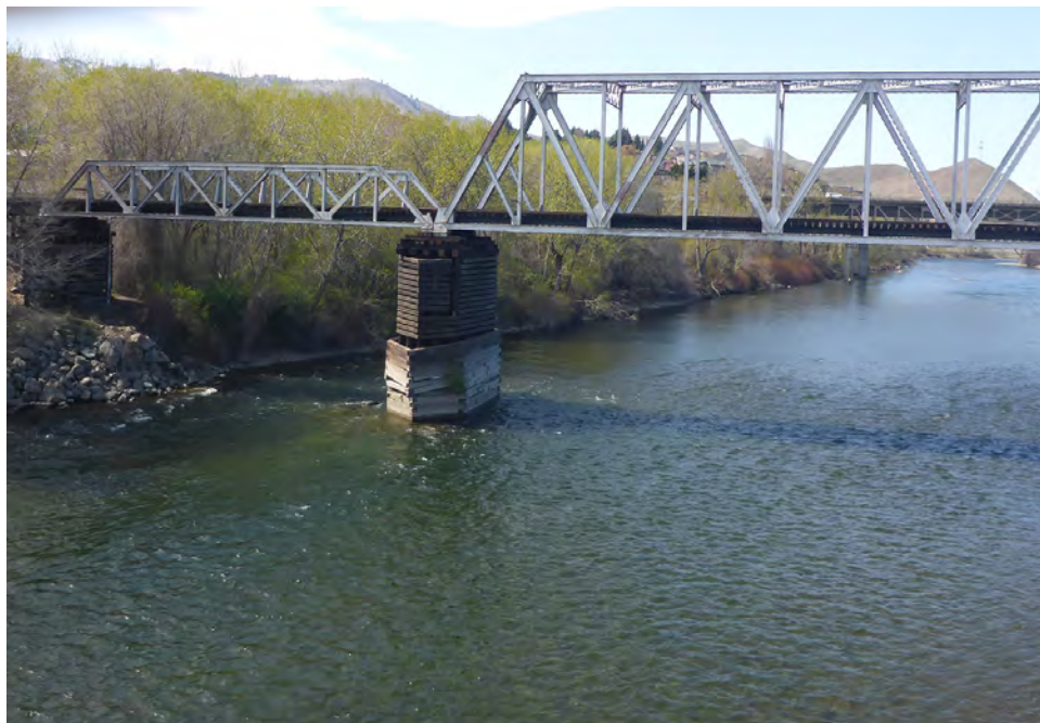
Wenatchee River Right Bank Upstream of Apple Capital Recreational Loop Trail Bridge
