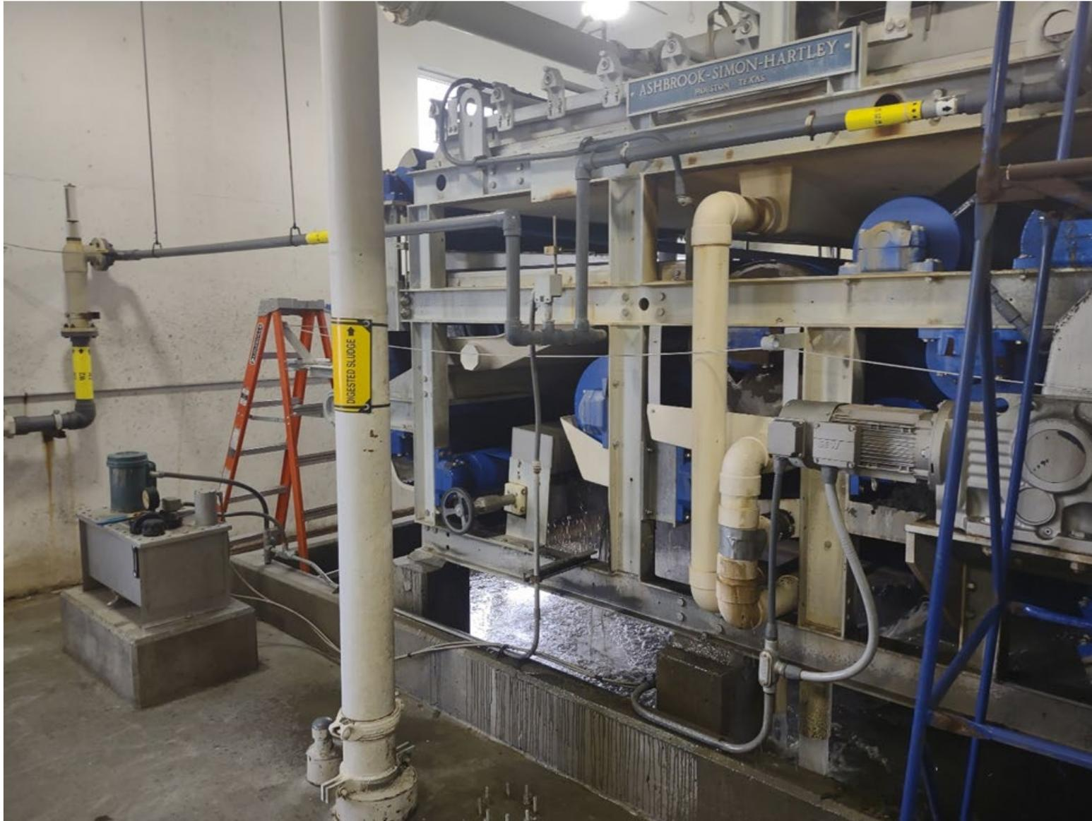
The biosolids are then scraped off the bottom belt and fall through the chute on the right into a dump truck below. The biosolids are now the consistency of Jello and are more easily transported to the drying beds for final processing.
