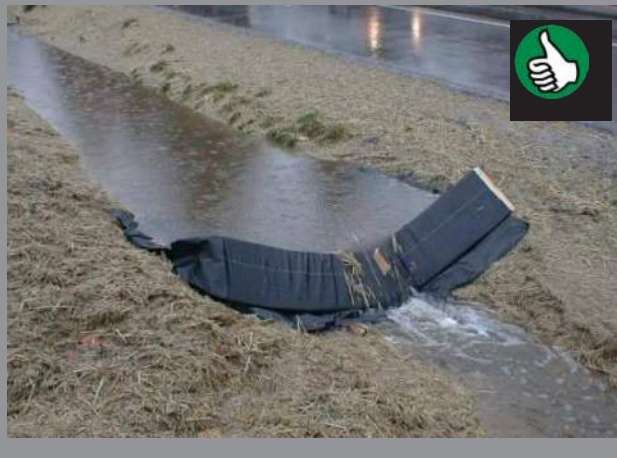
Good example of a properly installed check dam.
