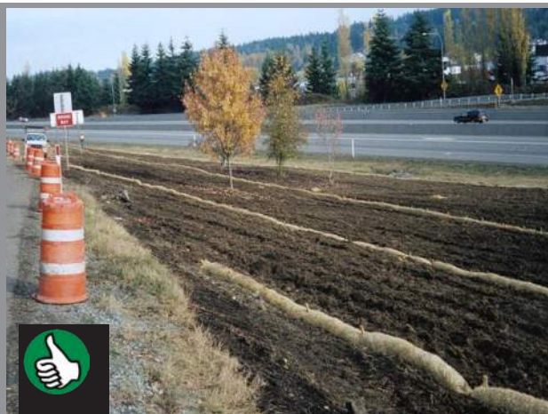
Good example of properly installed wattles.
