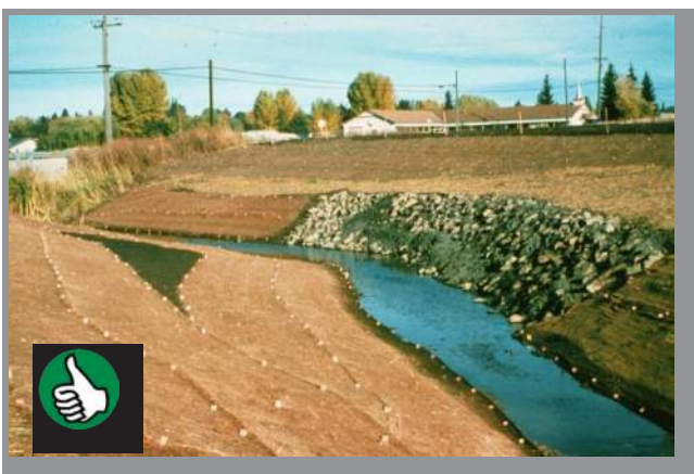
Stream stabilization with rock and coconut fiber erosion control blankets.
