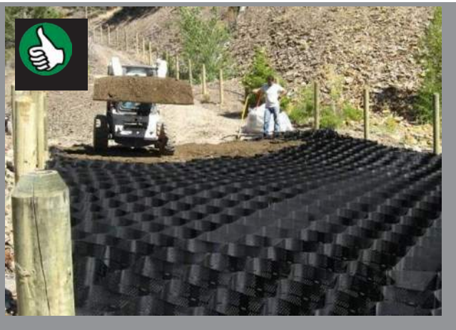
Example installation of cellular confinement system.
