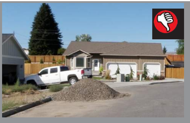
Stockpiles should not be stored in the street or on impervious surfaces that drain to street. Locate stockpiles away from drainage paths and storm drain inlets and protect against erosion. (Source: Douglas County)
