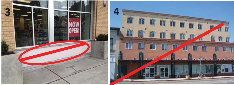
Figure E.6.1.e. Examples of acceptable and unacceptable use of EIFS. Buildings 1 and 2 mix EIFS with brick and other materials and integrate trim details around windows to add a sense of depth to the façade. Building 3 uses EIFS in between the window and sidewalk - this design is prohibited. Building 4 uses EIFS as the primary siding material, which is prohibited except in the North and South Wenatchee Business District areas.
