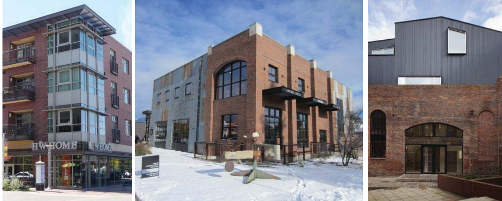
Figure E.6.1.c. Metal siding used appropriately in combination with other materials. The use of metal siding in each example above is secondary to masonry. The left and right images are more contemporary in character, whereas the middle image is more rustic and industrial, with more refined windows.
