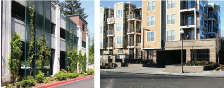
Figure 10.36.050(8)(b): The parking garage on the left includes decorative grillwork and vines to enhance its façade. The one on the right includes landscaping to separate the parking from pedestrians
