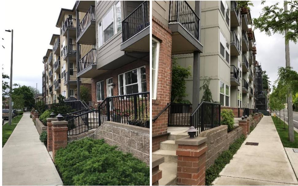
Figure C.1.c. The above images show ground-level residential frontages with setbacks of approximately 10 feet (left image) and 5 feet (right image) along different street frontages for this corner apartment building. These ground level units all have their own private unit access from the sidewalk and are elevated above the sidewalk to enhance the privacy to the units. The landscaping elements, brick posts, split-faced concrete block stoop walls, and black metal railings help to provide an attractive and effective transition between the public and private realm within the adjacent dwelling units.
