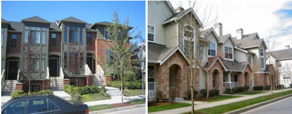
Figure E.3.1.c. The units in the left image each have distinct, but identical windows and roof forms. The outside unit on the right is differentiated through the use of building materials, window design, unit size, and façade detailing. The units in the right example include reverse elevations that add to the building's composition.
