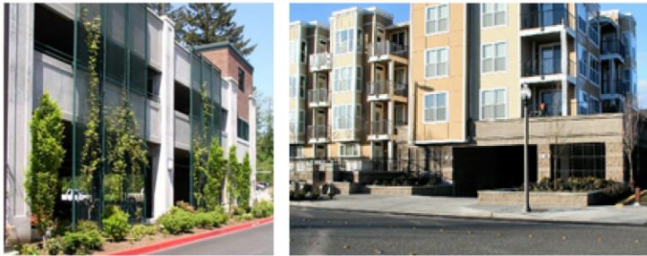
Figure 10.36.050(8)(b): The parking garage on the left includes decorative grillwork and vines to enhance its façade. The one on the right includes landscaping to separate the parking from pedestrians
