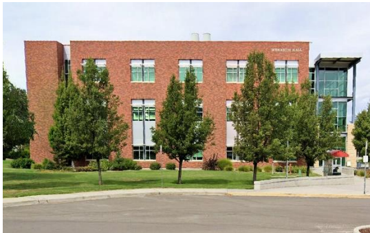
Figure 10.36.050(3.2). Seen from a proper distance, a building 0.8 times viewing distance will appear as an individual element within its surroundings. Even though the main façade is uniform, it does not feel too dominant. Note that the articulated corner, the articulated entry and the other building elements plus the amount of window area make the building more interesting and seem “friendlier”. Also note the way the trees reduce the building’s visual impact.
