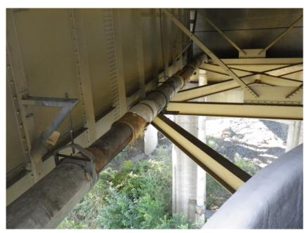
WSDOT during routine bridge inspection and limited observations from the north bridge abutment, both have degraded and, at a minimum, replacement of the insulation and heat tape is necessary.
