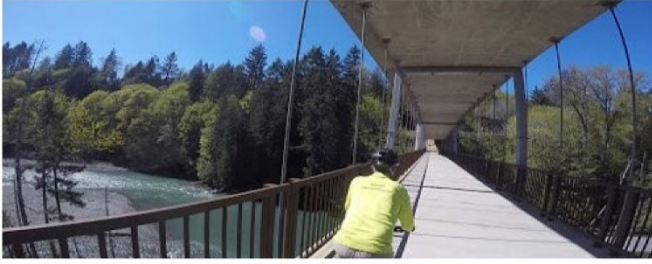
Hanging Pedestrian Bridge
