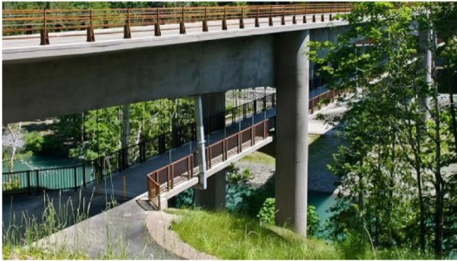
Elwha River Bridge, WA - Combined Bridge
