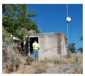
cracked in multiple places. The inside of the structure has a dirt floor with poor access conditions due to a grade separation. Additional valve hardware is present in an external, substandard vault adjacent to the structure. The 16 inch pipe between the valve vault and the reservoir has experienced failure in the past due to corrosion and its condition entire is suspect.
