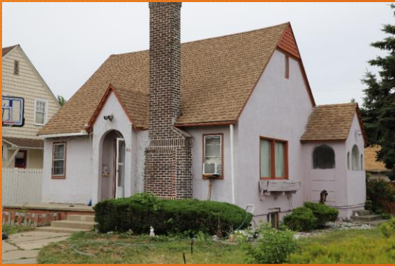
Jones House, 900 S Highland
