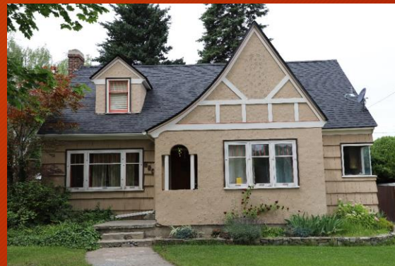
McBeth House, 920 S Highland
