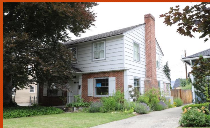
Garrison Revival 937 S Highland (1938)
