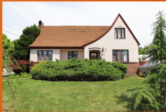
Schroeder House, 901 S Highland
