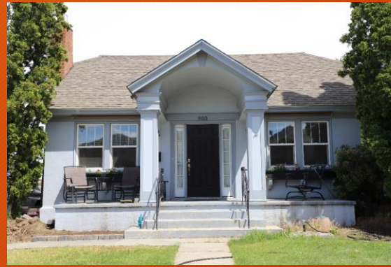
Hilt House, 903 S Highland
