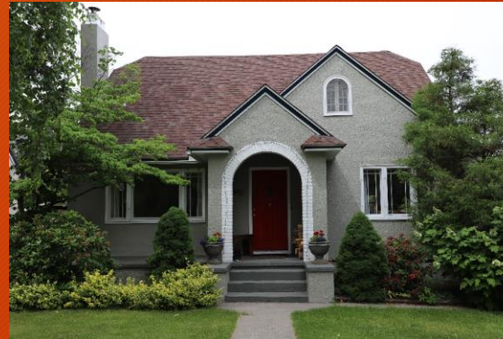
Battey House, 912 S Highland
