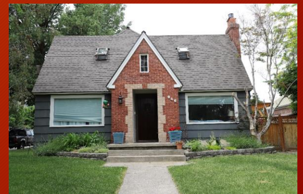
Kemp House, 946 S Highland
