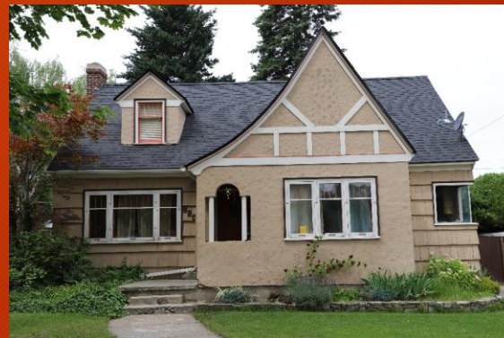
McBeth House, 920 S Highland
