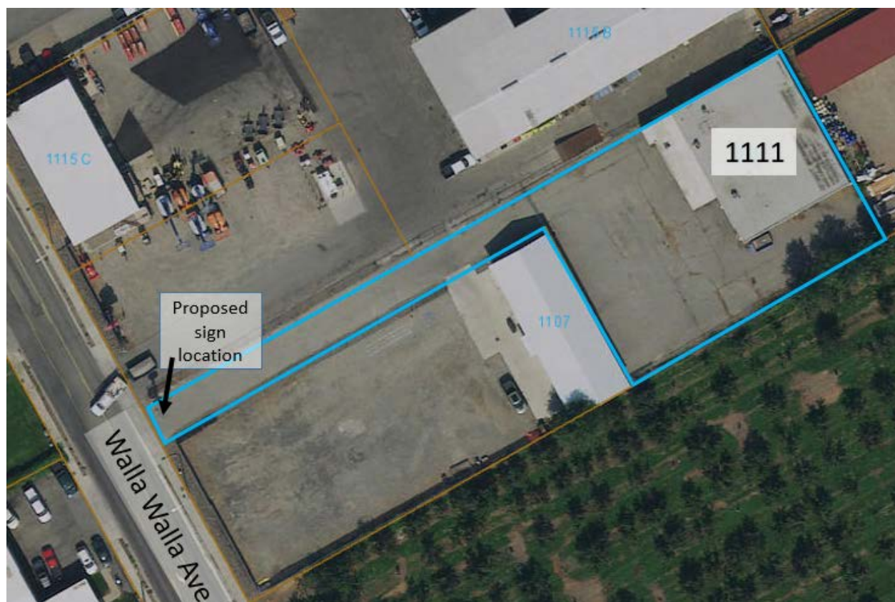
Figure 1. Aerial image of proposed project
