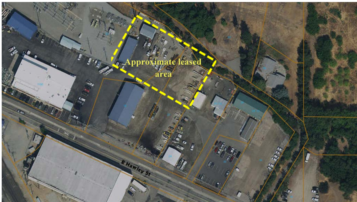
Figure 1. Aerial image of proposed project
