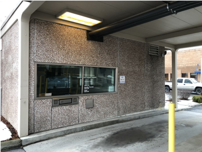
Under car port (North side)
