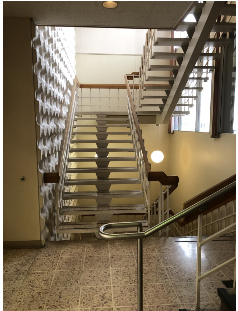
Interior staircases from main floor landing.
