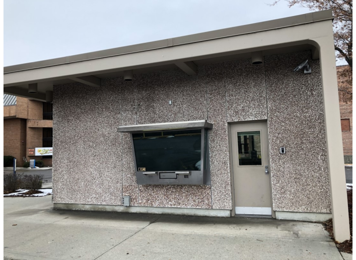
Orondo Ave. side (South)
