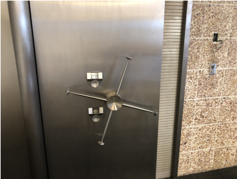
Vault doors, safety deposit box vault, private customer room
