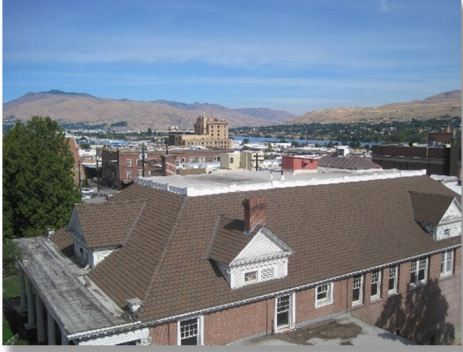
Sloped roof with asphalt shingles
