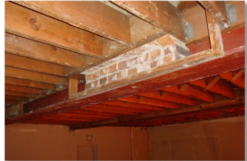
Masonry chimney bearing on steel beam
