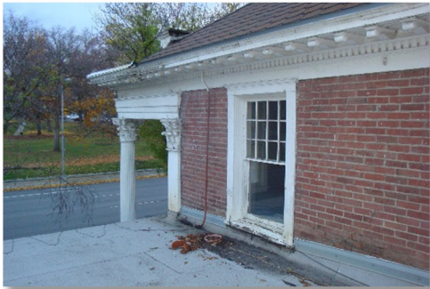
Sill of tall window close to roof
