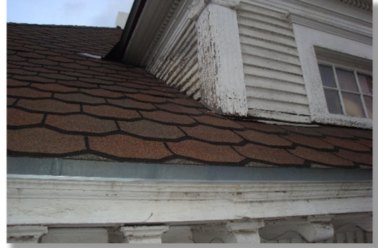
New asphalt shingles to mimic existing 'fish scales'
