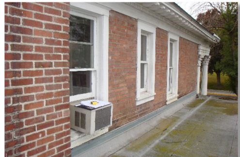
Other window sills raised above roof (north)
