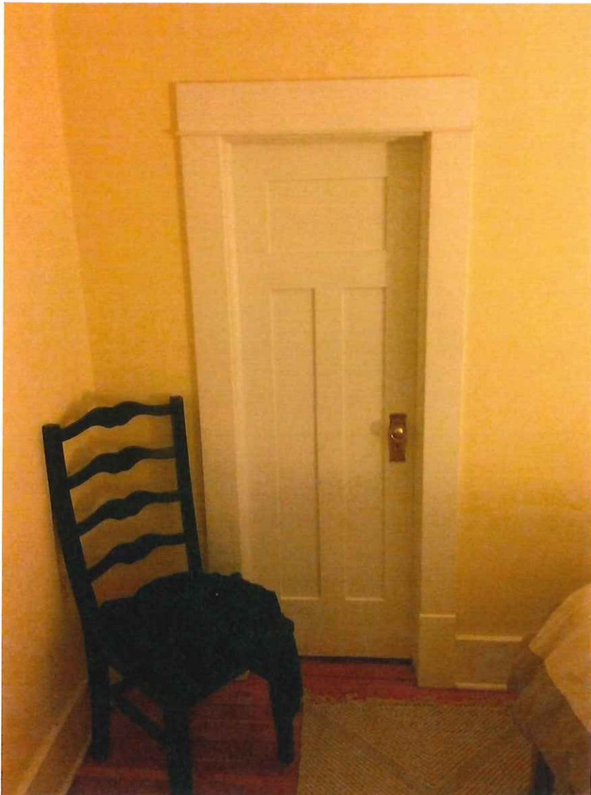
Figure 2 –Typical 2-Panel Interior Door inside house (included for reference)
