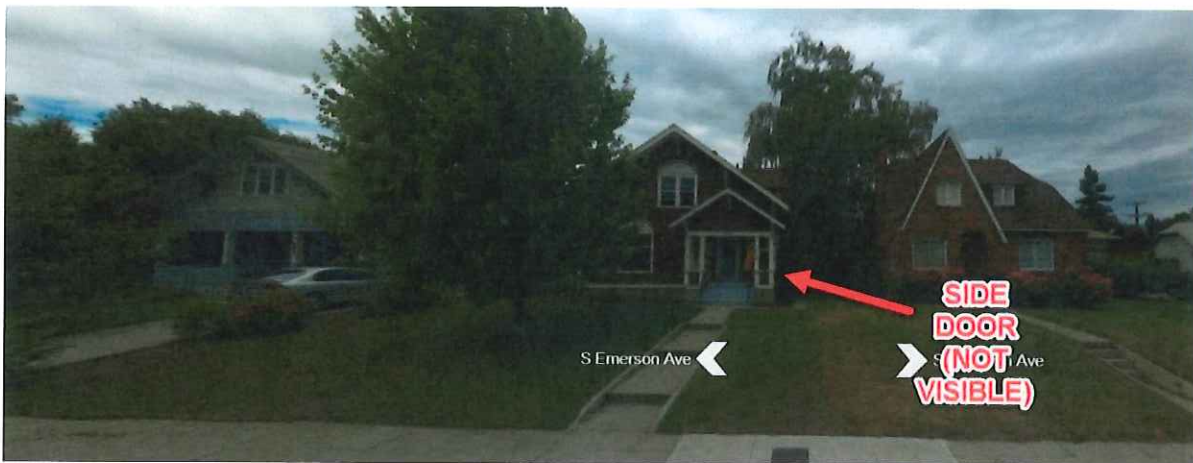
Figure 6 – Front View looking west showing General Location of Side Door (Image Source: Bing Streetside)
