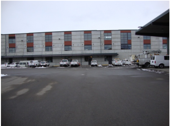
N side of Building 1 – Partially Covered Parking
