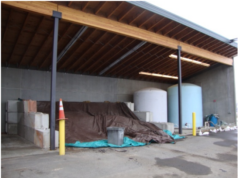
Cold Mix & Deicer Storage (Bldg. 5)
