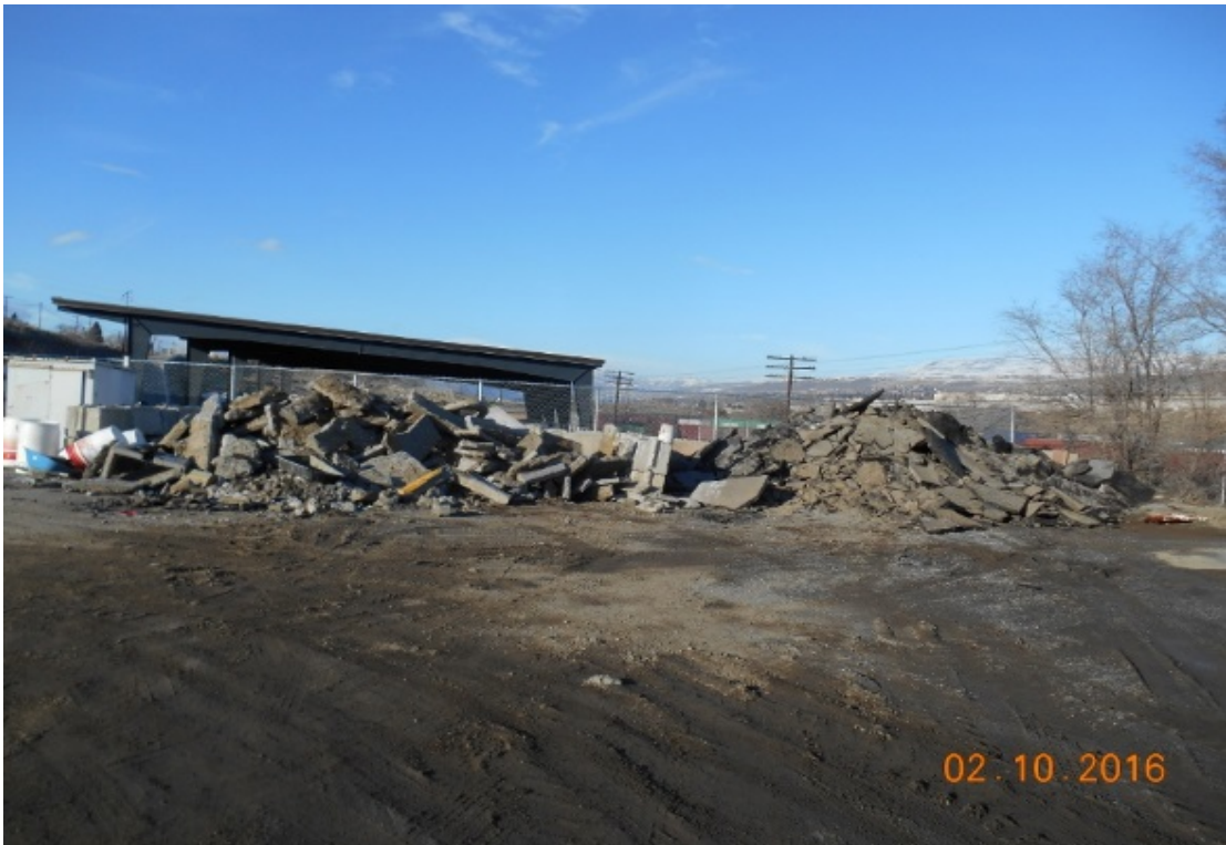
Asphalt and concrete debris storage – NE corner
