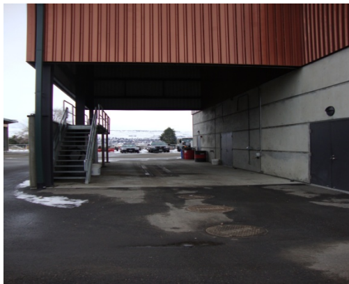
Vehicle Wash Bay (N of Bldg. 3)
