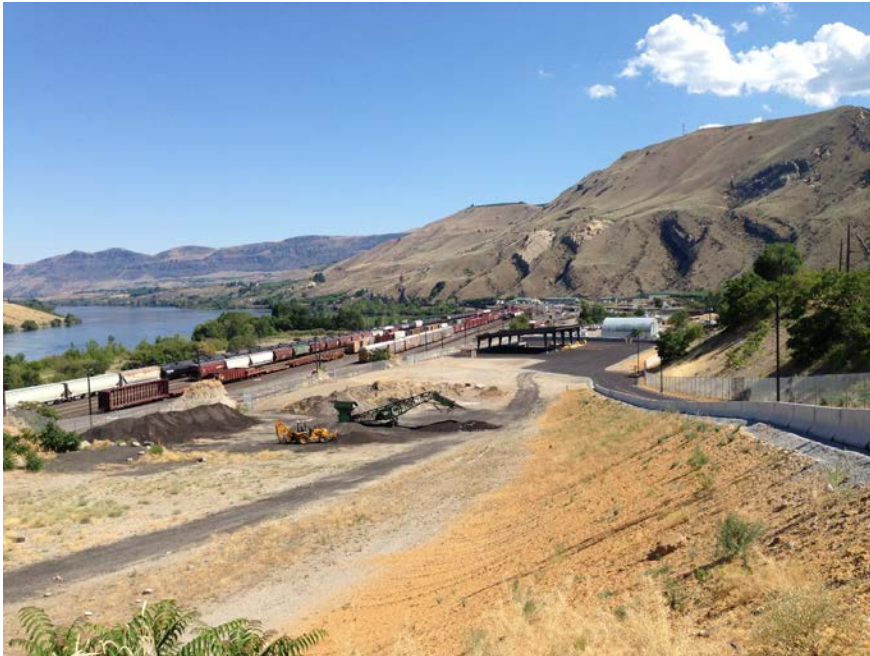
Asphalt debris storage – North corner
