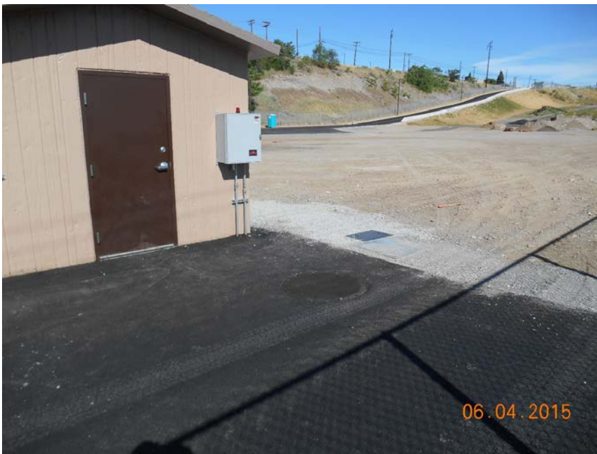
North of Decant Facility
