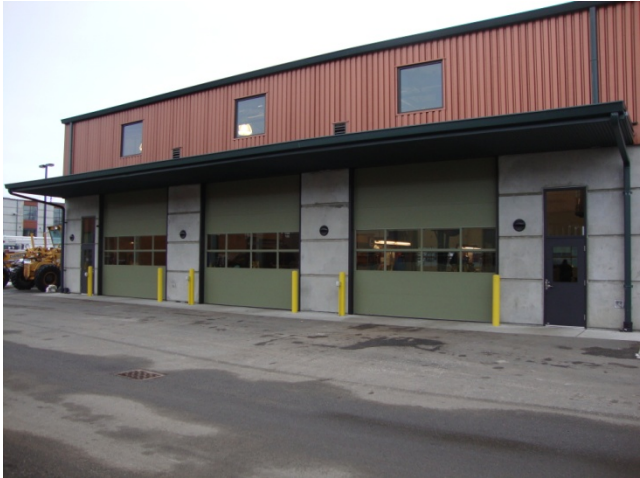
Building 3 – Fleet Maintenance & Repair Shop
