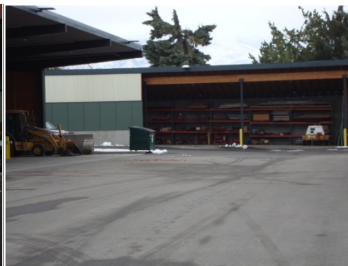
Cardboard Recycling (N end of Bldg. 2)
