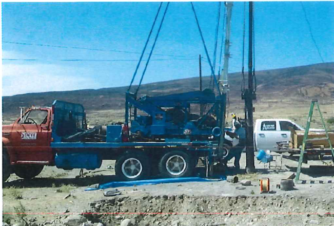
Cable Tool Drilling Rig
