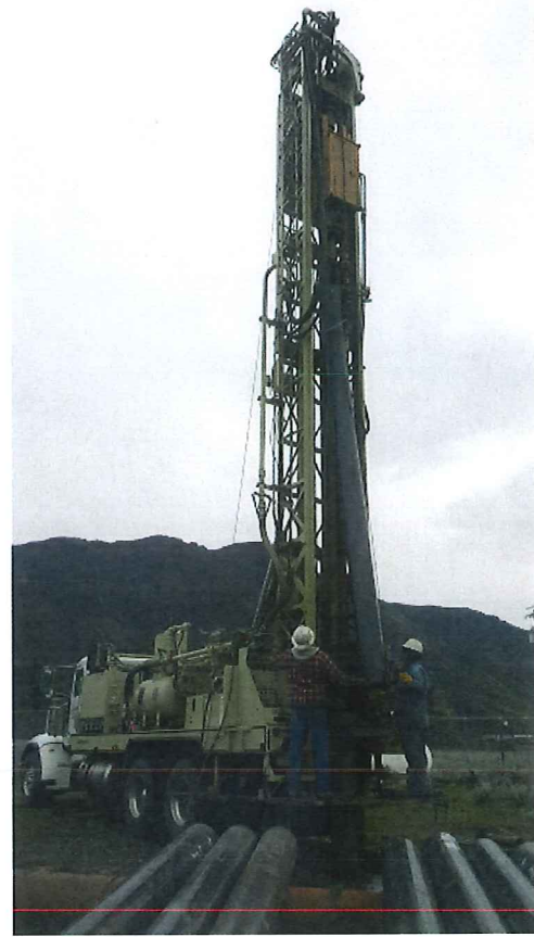
Rotary Drilling Rig
