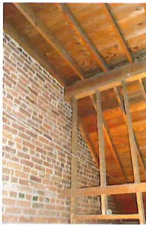
Exposed brick wall
