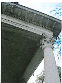
Porch soffit & cornice
