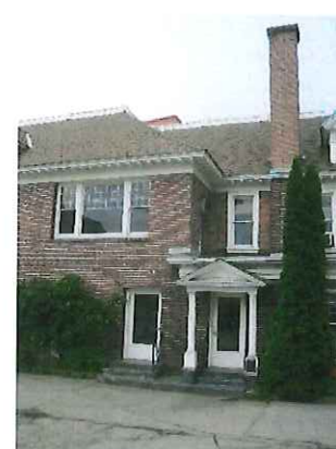
No ramp at main entry
