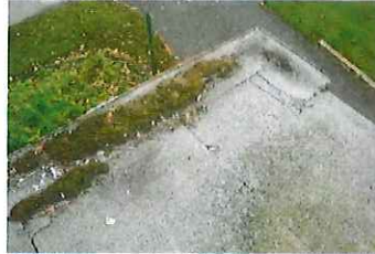
Clean moss & debris
