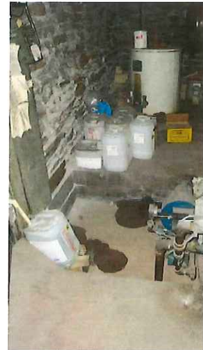
Floor & equipment demo
