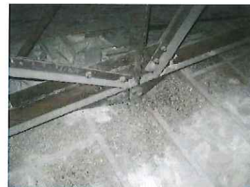
Exposed steel truss connection
