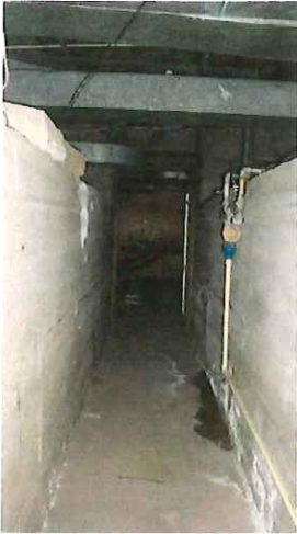
Wall & floor demo
